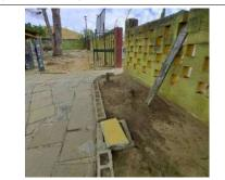
Defect Description: Water valve chamber is filled with debris and missing cover.
