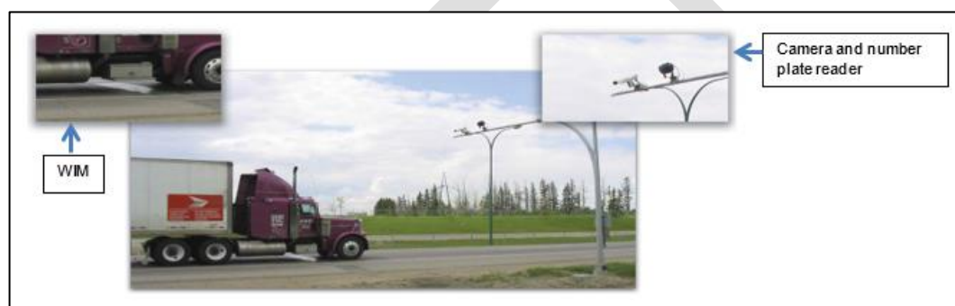
Figure 10-4: Typical VWS site
