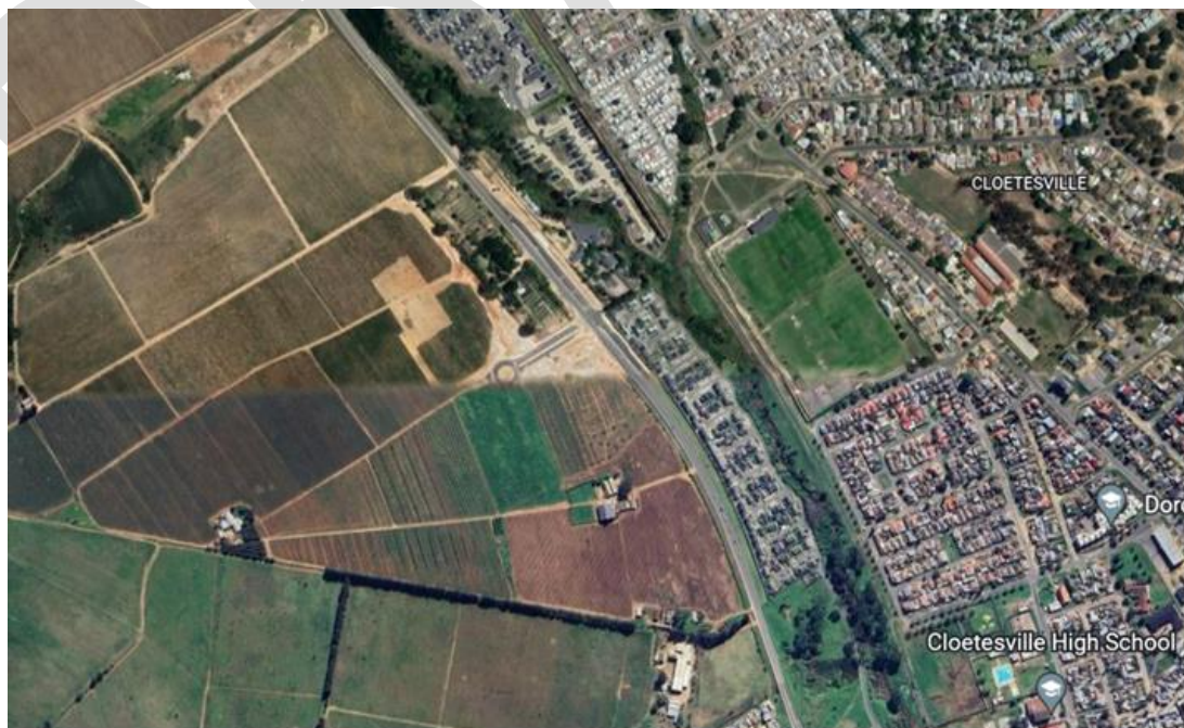
Figure 7-5: Current access construction and dualling of the R304 to provide access to Newinbosch (Precinct 10 of proposed Adam Tas Corridor development – just west of the R304 and northwest of Kayamandi)
