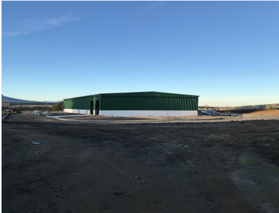
New MRF building under construction
