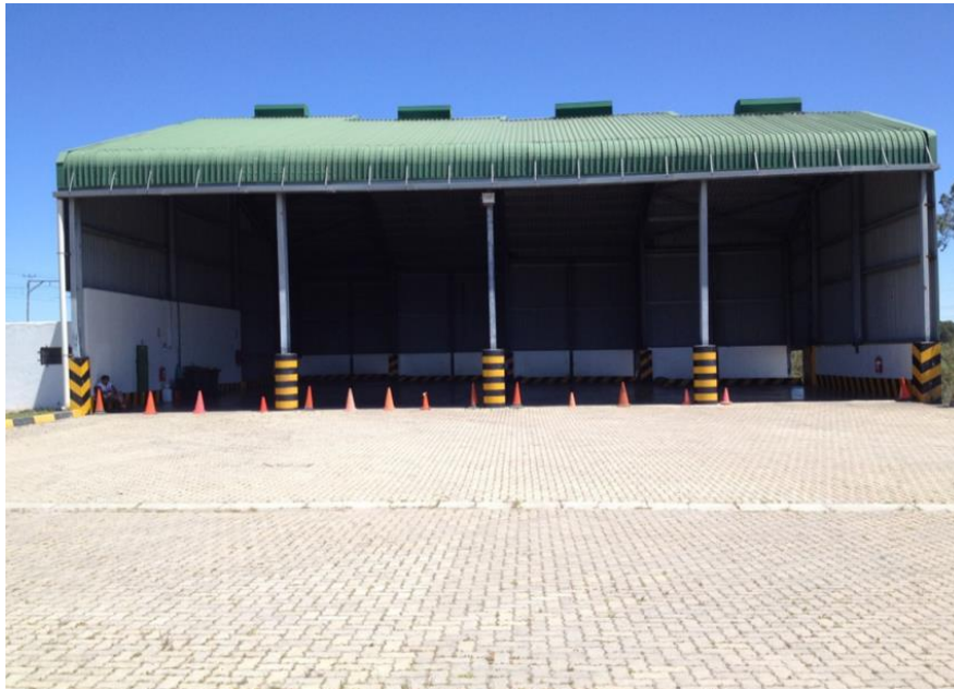
Klappmuts Transfer Station waste reception apron
