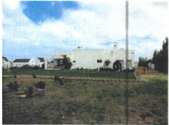
Location of Portion 1 in foreground in relation to existing dwelling
