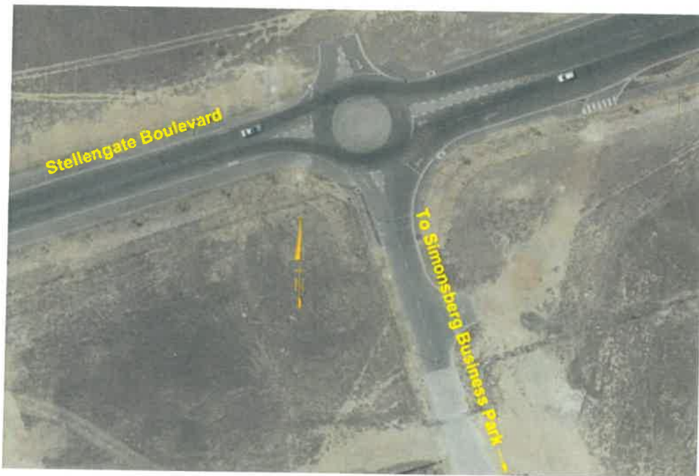
Photo 2 : Existing Stellengate Boulevard/Simonsberg Business Park Access intersection lane layout
