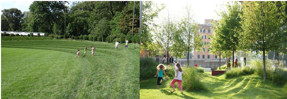
Figure 62 - Examples of stormwater detention areas designed to be used as recreational spaces in times when its not raining
