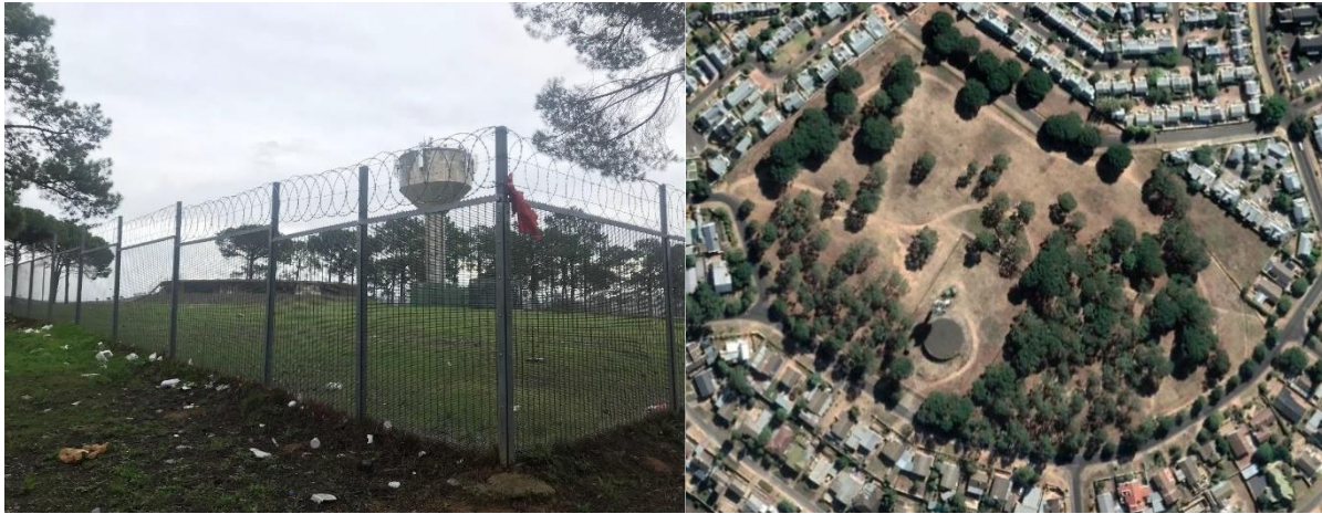
Figure 55: Water reservoir and tower
