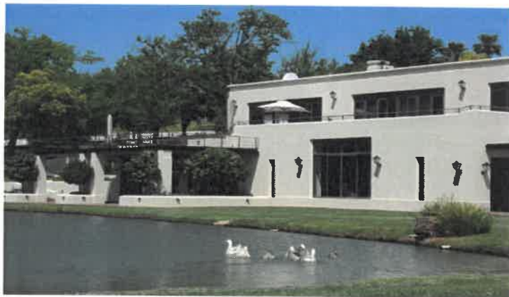
Figure 5 wine cellar/ restaurant and conference facility
