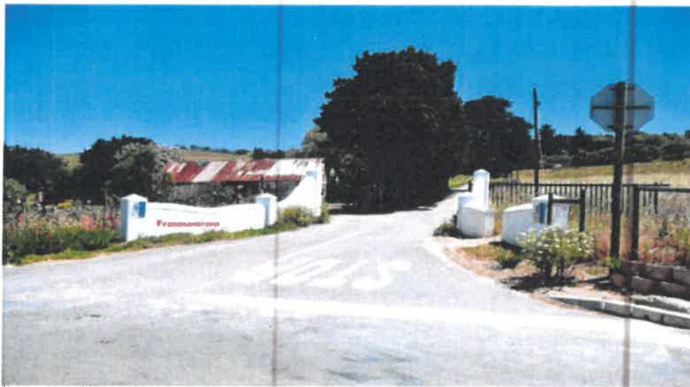
Farm entrance off Vlotenburg Road
