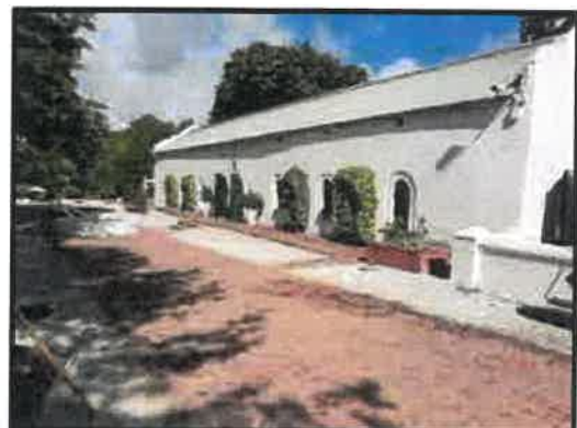
Photo 16: Side of Original Cellar used for Wine Tasting
