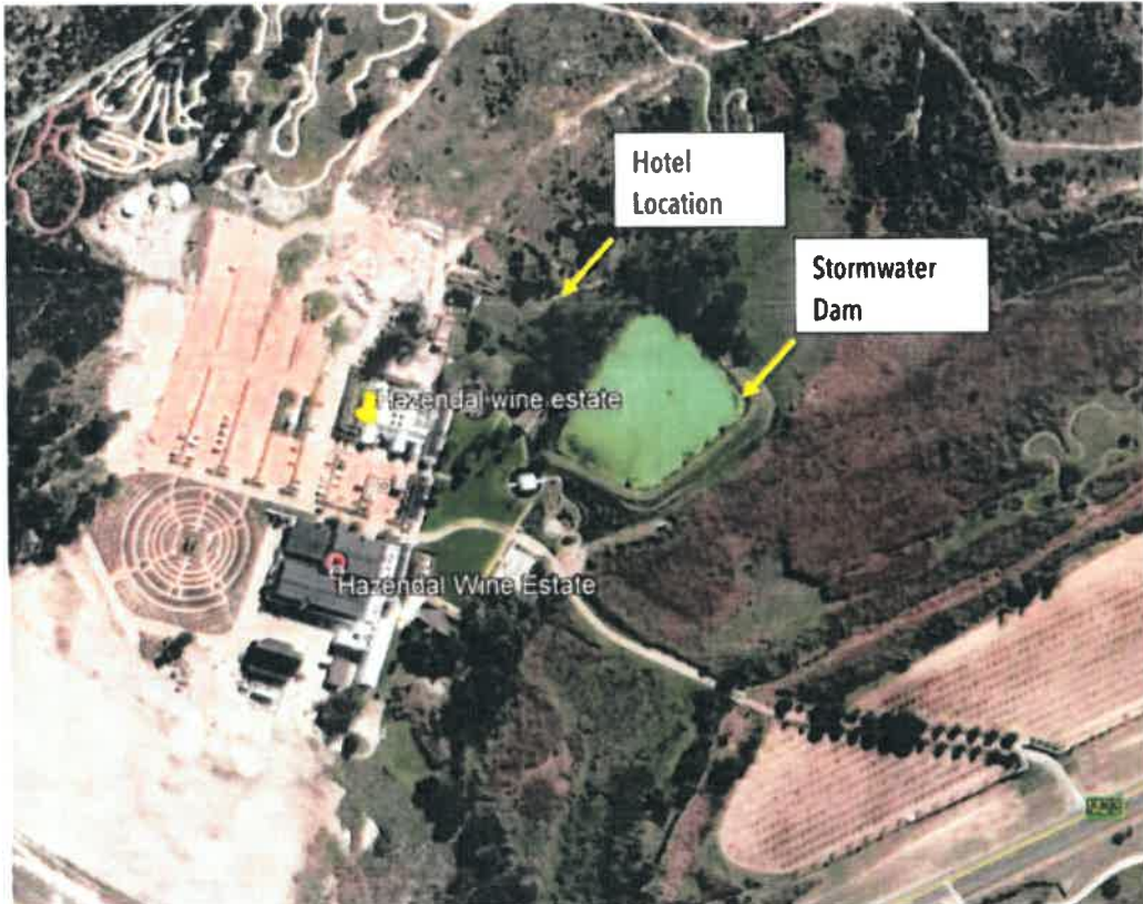
Figure 4-2 Aerial image of pond location
