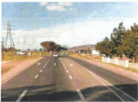
Photo 1 Bettelary Road Eastbound View towards Kruis Street
