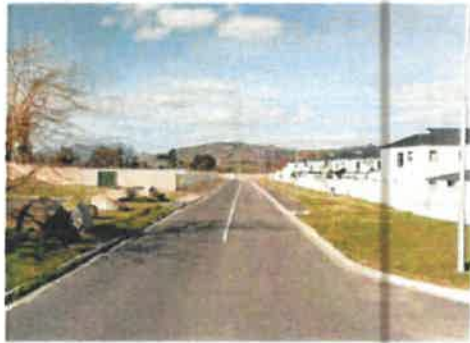
Photo 4 Ronelle Street Eastbound View towards Schoongezicht
