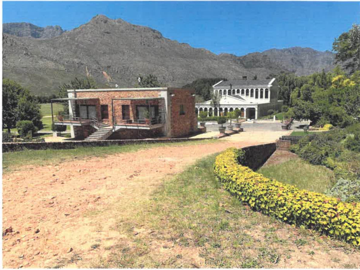
Building situated in the south western corner comprising residential apartment suites at first floor level and four garages at ground floor level
