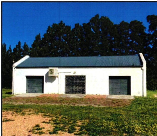
The farm store building
