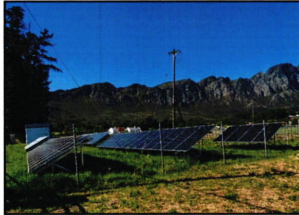
Solar panel installation
