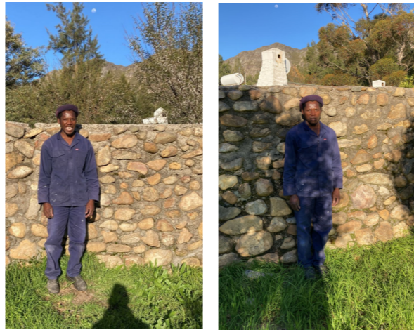
Photos indicates existing wall height variants.
