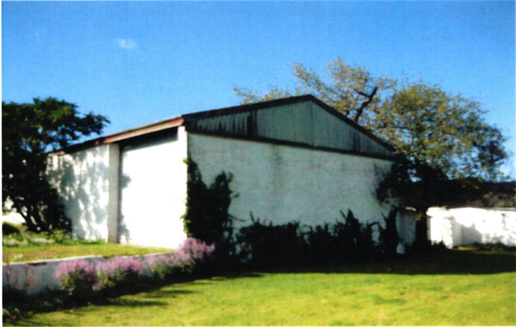
Farm building on farmstead
