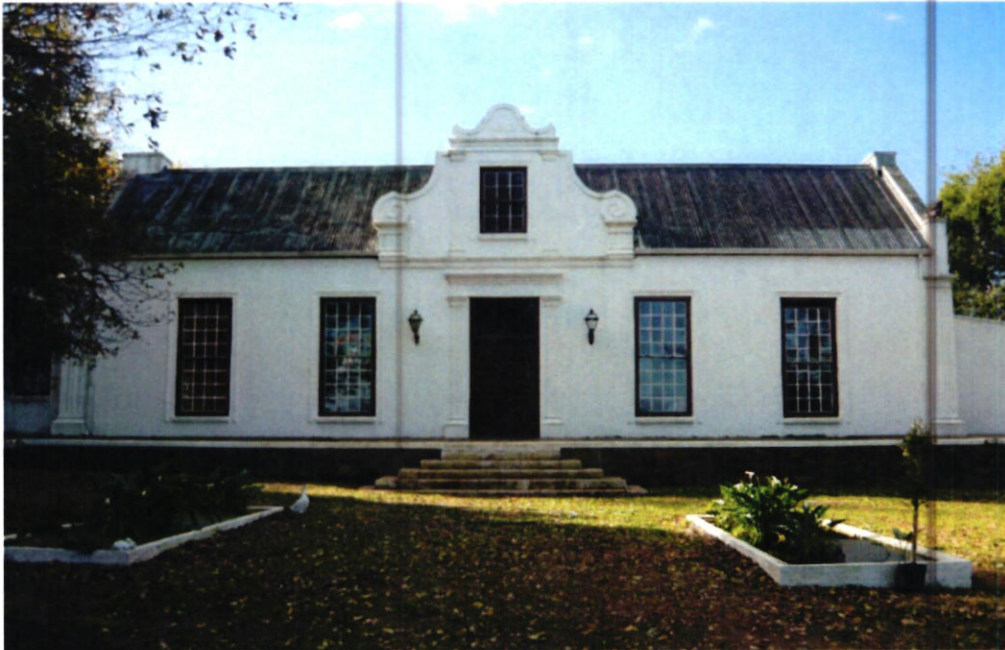
Existing Manor House
