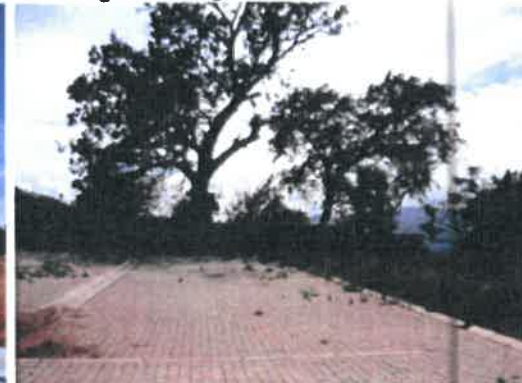
Internal road on Mentoor Estate to connect
