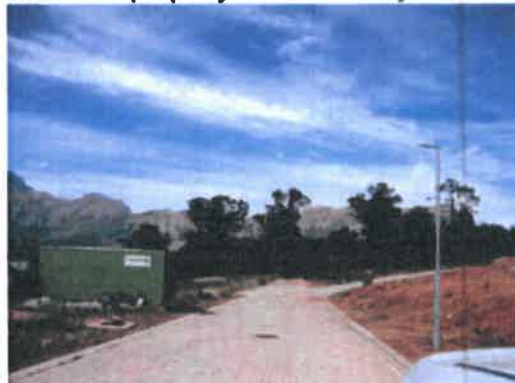
Existing access road to be extended
