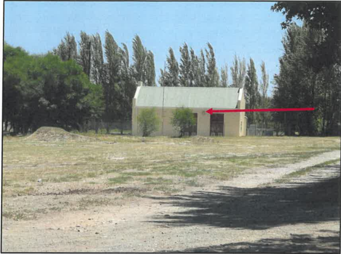
Photo 3: View of the pump station on the adjacent Leopards Leap property, 2019
