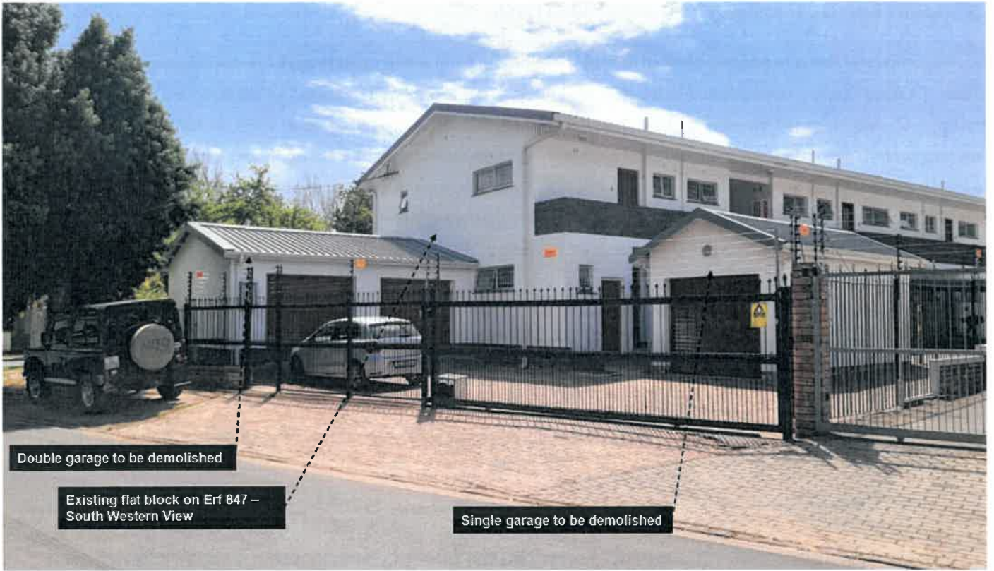
Figure 5: View from the Southwest (Koch Street) of the existing flat block on erf 847
