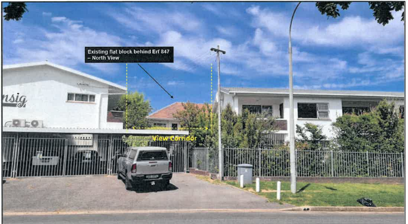
Figure 6: View from the North that shows the view line from the flat block located behind the application site
