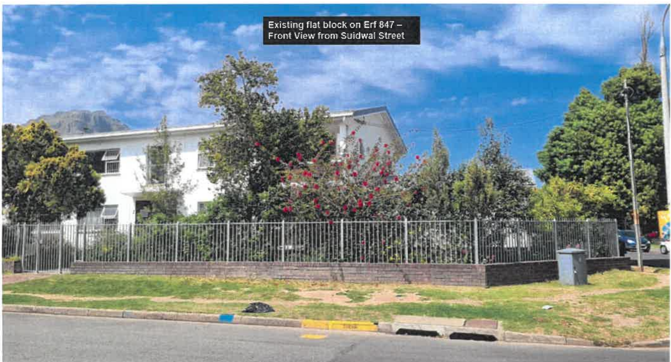
Figure 4: View from the North (Suidwal Street) of the existing flat block on erf 847
