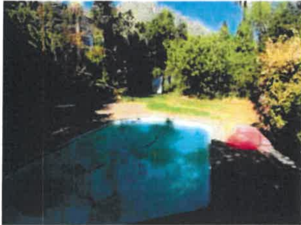
Existing pool to be demolished
