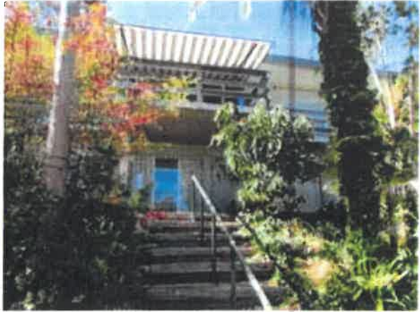
Existing dwelling as viewed from rear garden
