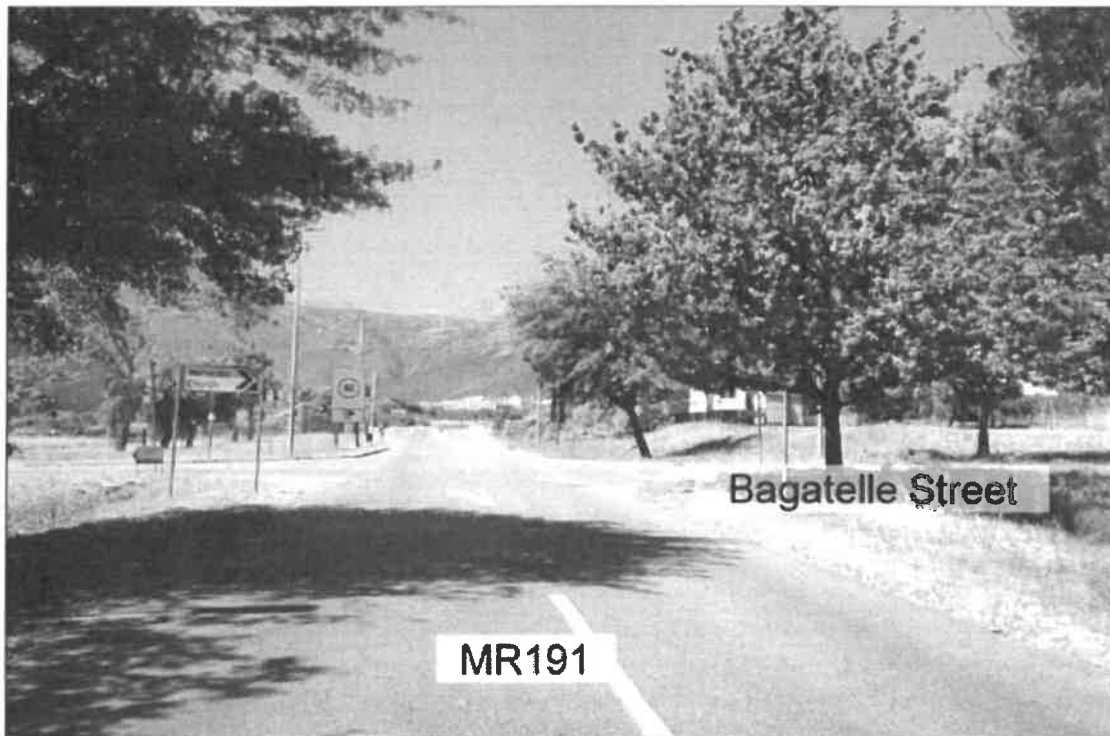
Figure 4: Affected Roads – street view
