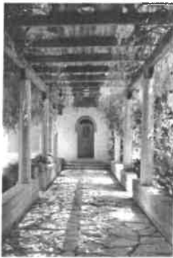
Figure 23: Covered walkway servicing as noise screening device
