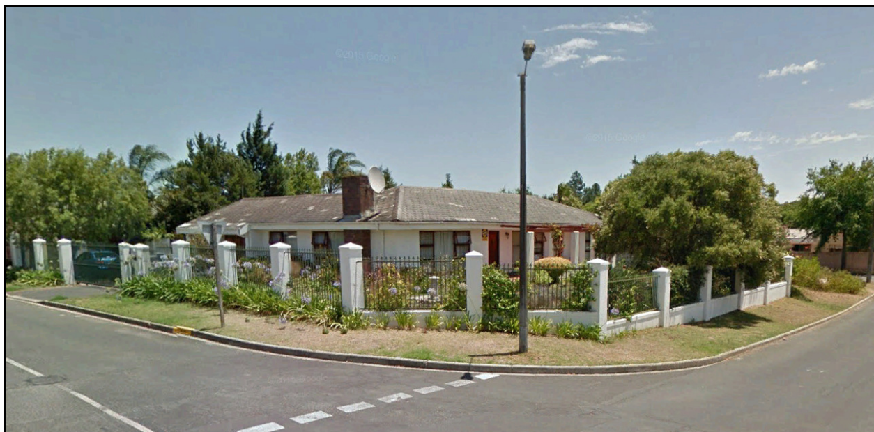
Figure 2: Existing dwelling at 2 Sultan Street
