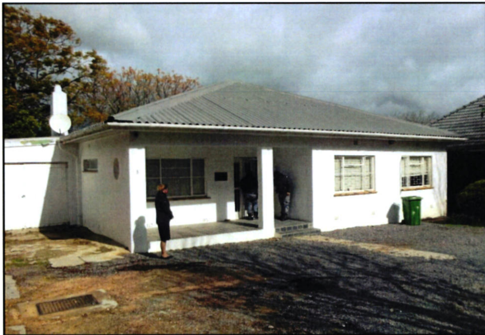
Front view of the building on Erf 425
