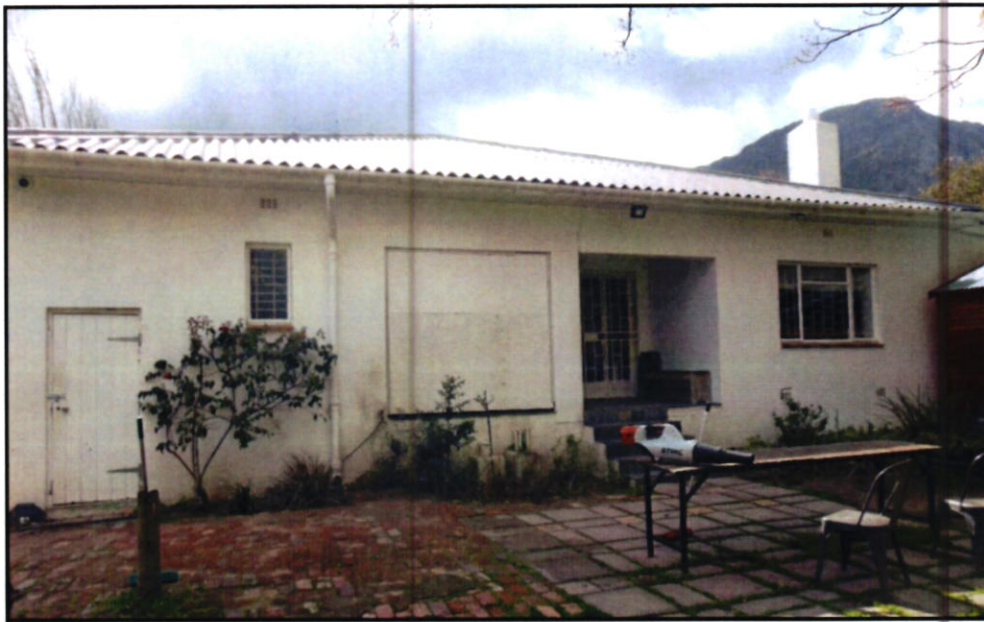
Rear view of the building on Erf 425
