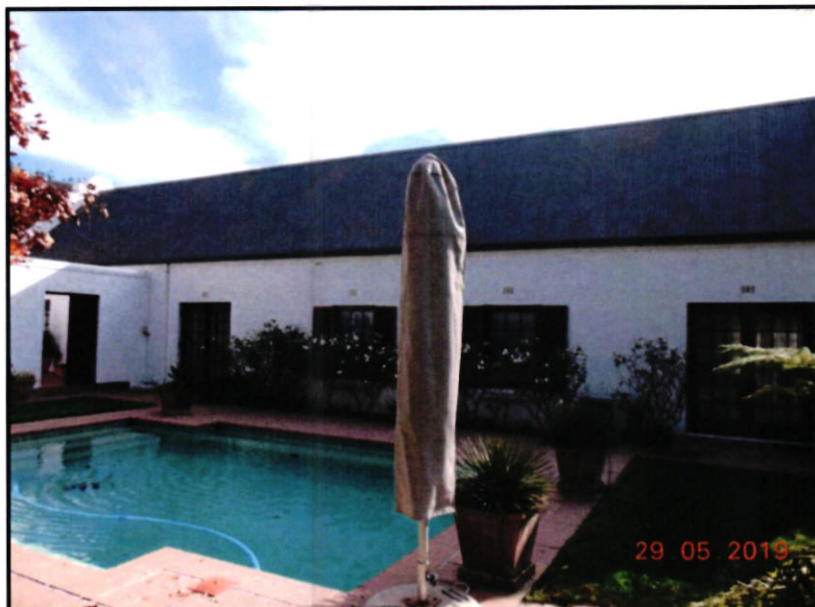
Portion of the buildings containing one of the approved guest suites consisting of two bedrooms with a guest pool in the foreground
