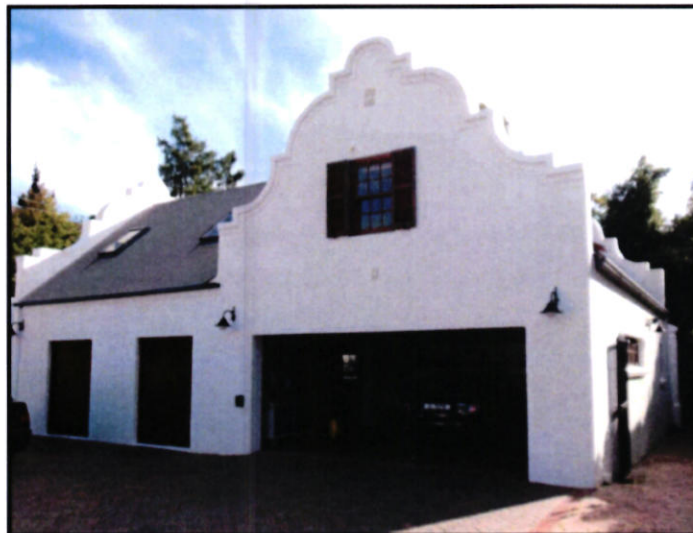
Outbuilding containing Garage, Laundry and first floor Guest Unit
