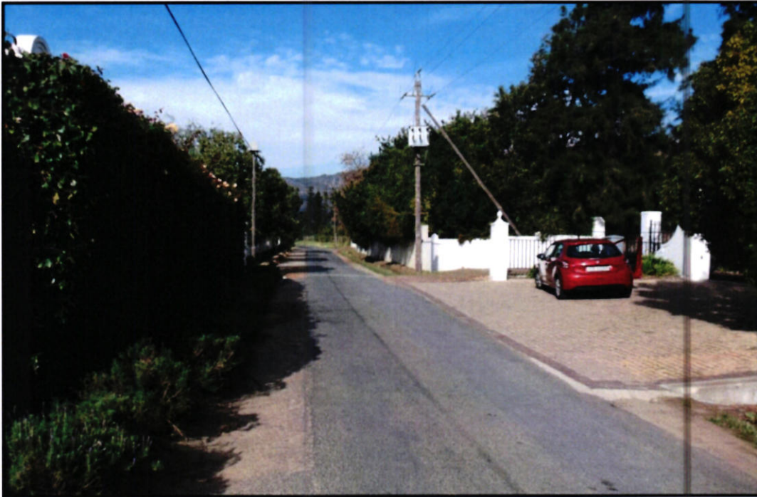
Sight distance in an easterly direction from the entrance gate
