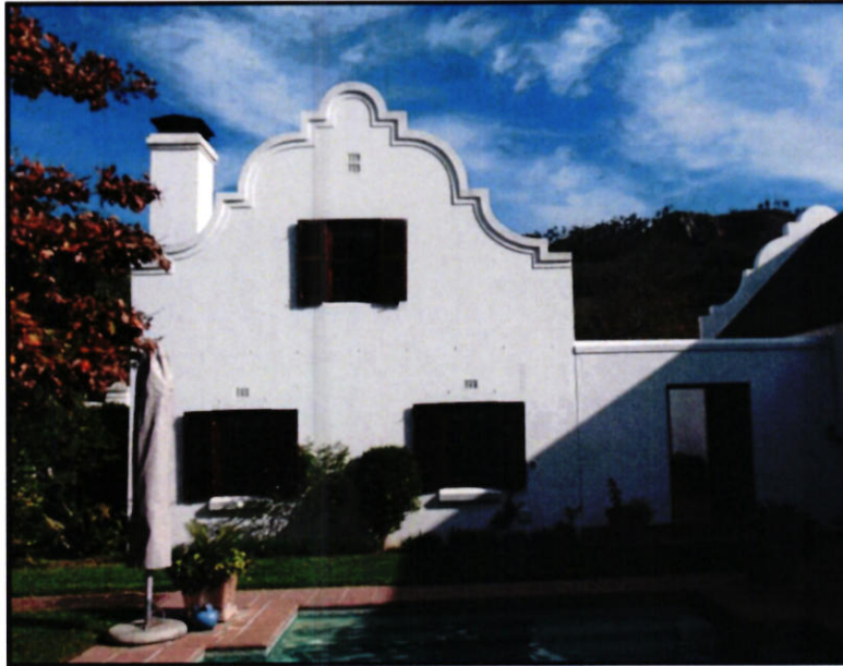
Double story section with living room downstairs and bedroom above which makes up a portion of the second guest suite
