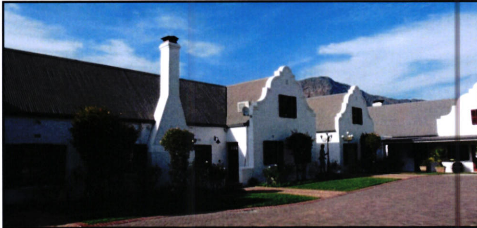
Section of the buildings containing proposed guest facilities on the ground floor
