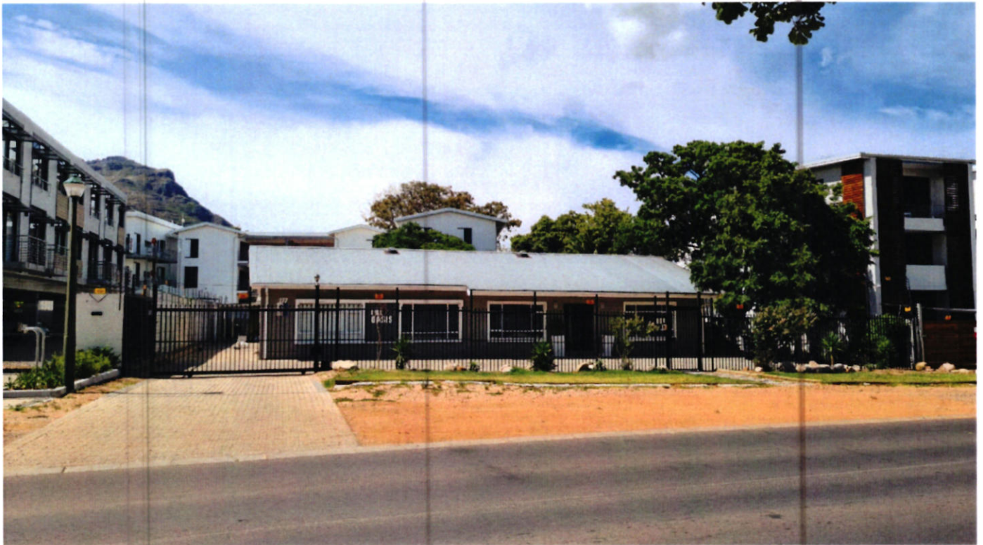
Figure 4: Existing single storey building on site.
