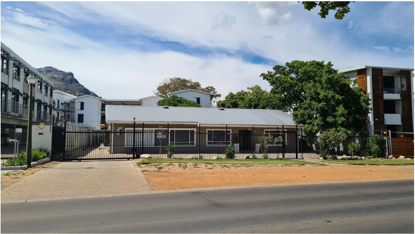
Figure 4: Existing single storey building on site.
