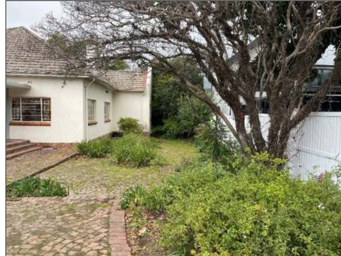
2) Right hand side of main building
