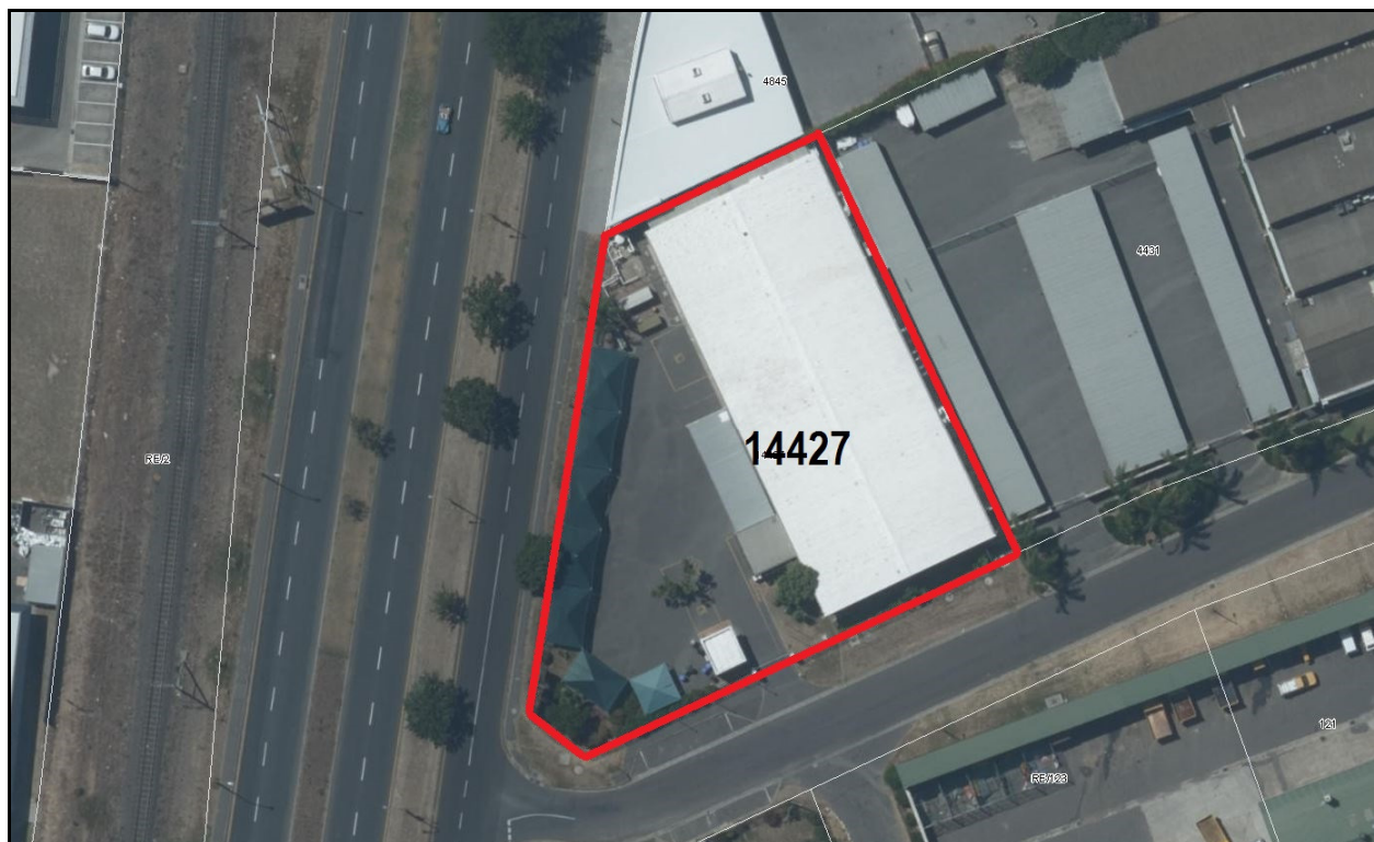
Figure 2: The existing building on Erf 14427, Stellenbosch
