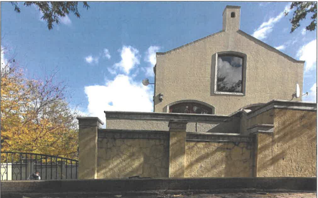
Figure 6 Eastern Elevation of the Existing Dwelling House
