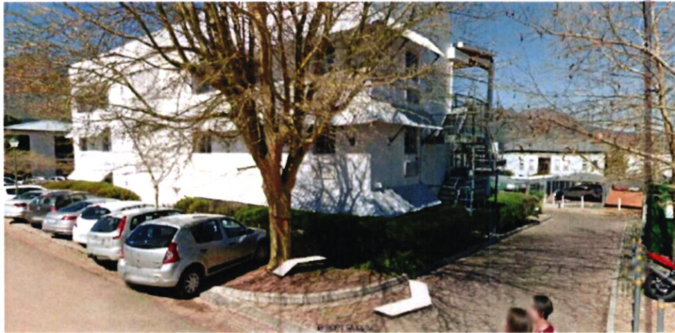
Photo 1: View of Quantum House where Limitless Acton Academy is proposed to accommodate the ground floor. The entry access road to the property can be seen on the foreground.
