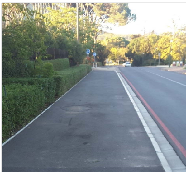
Figure 26: Stellenbosch town: Good example of a shared facility for pedestrian and cyclists that is of sufficient width (Marais St)
