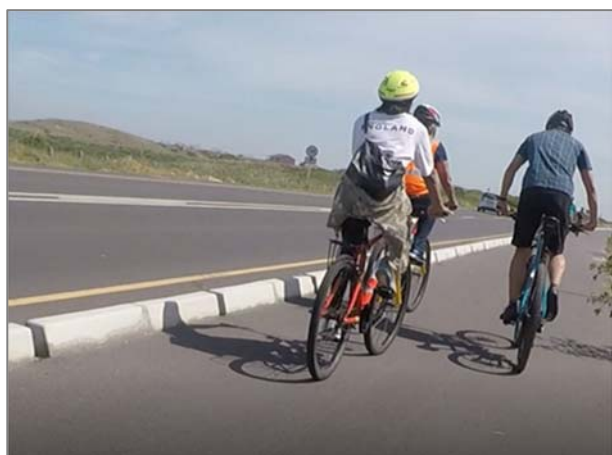
Figure 68: Local example of delineated kerb separation (R27 towards Melkbosstrand)
