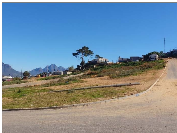
Figure 36: Groendal/ Langrug: Road infrastructure for future housing development lacks infrastructure for walking and cycling
