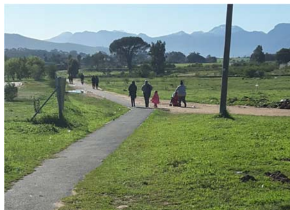
Figure 25: Klappmuts: Off-road NMT facility provided but lack of lighting and insufficient width
