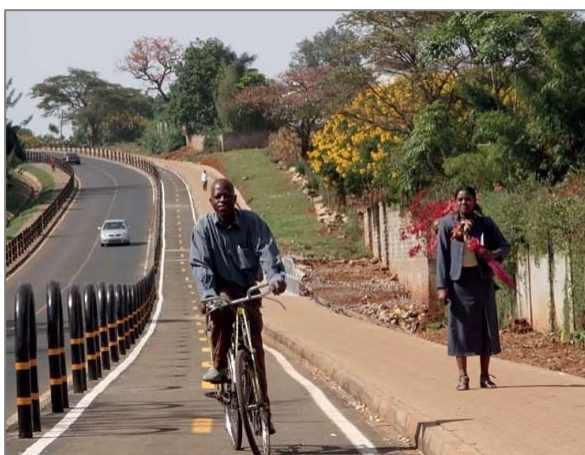
Figure 67: Physical separation between a bi-directional bicycle route and the roadway (Example: Nairobi in Kenya)
