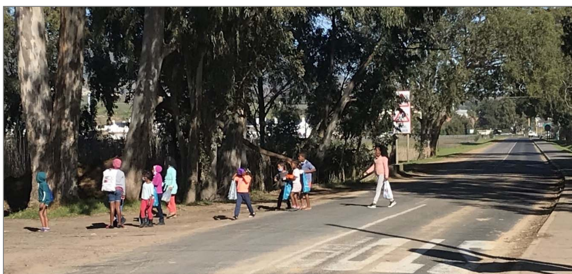
Figure 15: Koelenhof: Lack of safe crossing opportunity along desire line to/ from local school
