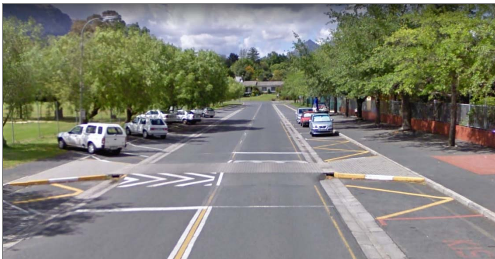
Figure 43: Krigeville: Example of a existing raised pedestrian crossing in front of a school
