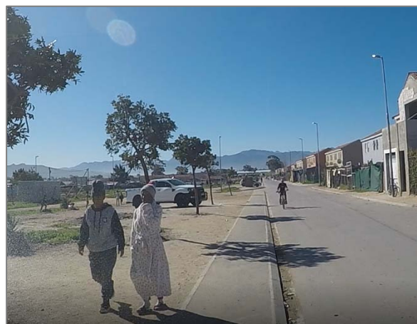
Figure 37: Klappmuts: Provided sidewalks are too narrow
