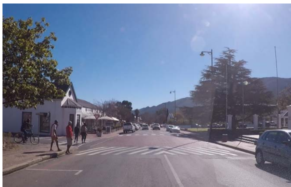
Figure 5: Franschhoek: Raised pedestrian crossing in CBD
