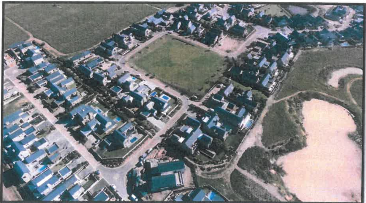
Figure 6: The Longlands residential estate (abutting the subject property)
