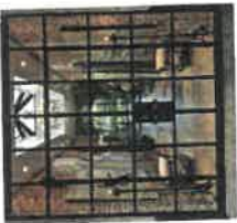
EXAMPLE OF TYPE OF PROPOSED REINFORCED INFL. GLAZING BEHIND EXISTING GARAGE DOORS AND FOR NEW OFFICE DOORS
