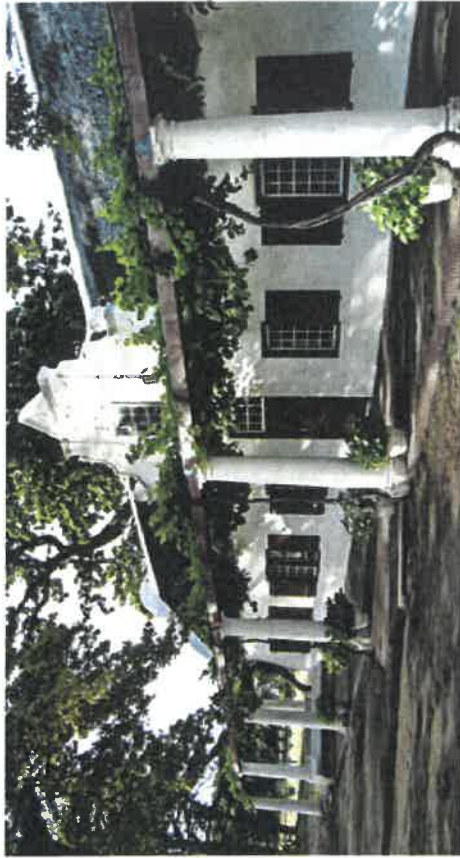
4.1.2 Front elevation of the T-shaped homestead
