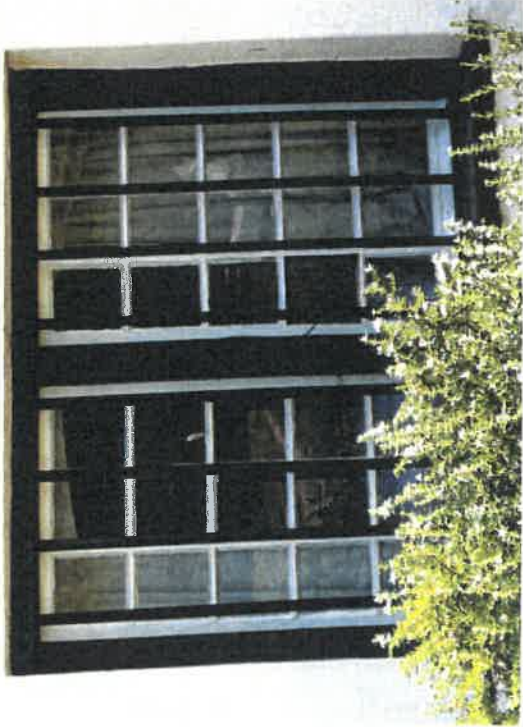
4.2.5 Typical double casements c 1912
