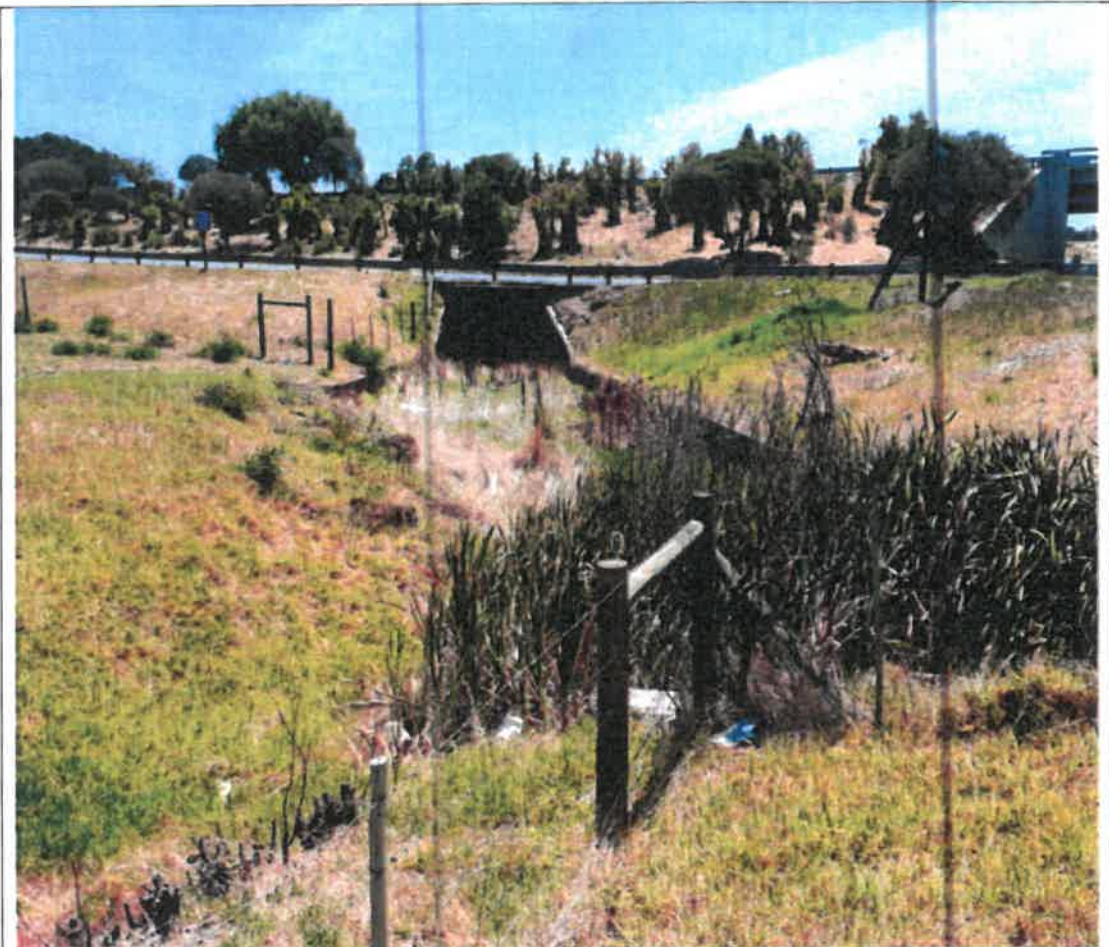
FIGURE 3: N1 PIPE CULVERT
