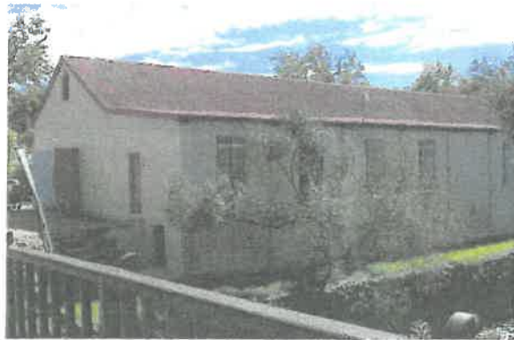
PHOTO 5: VIEW FROM PEDESTRIAN BRIDGE
