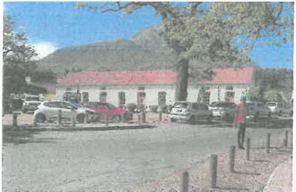
PHOTO 4: VIEW FROM CORNER OF PASTORIE STREET AND THE AVENUE (DIE LAAN)
