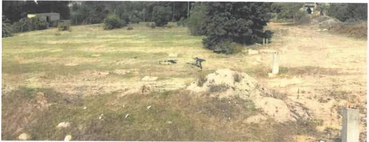
Photograph 6: Remnants of earlier building-works excavations and unfinished columns
