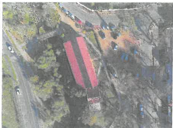
PHOTO 8: AERIAL VIEW OF LEASE AREA 1 AND LEASE AREA 2 OVER ERF 2751, STELLENBOSCH
