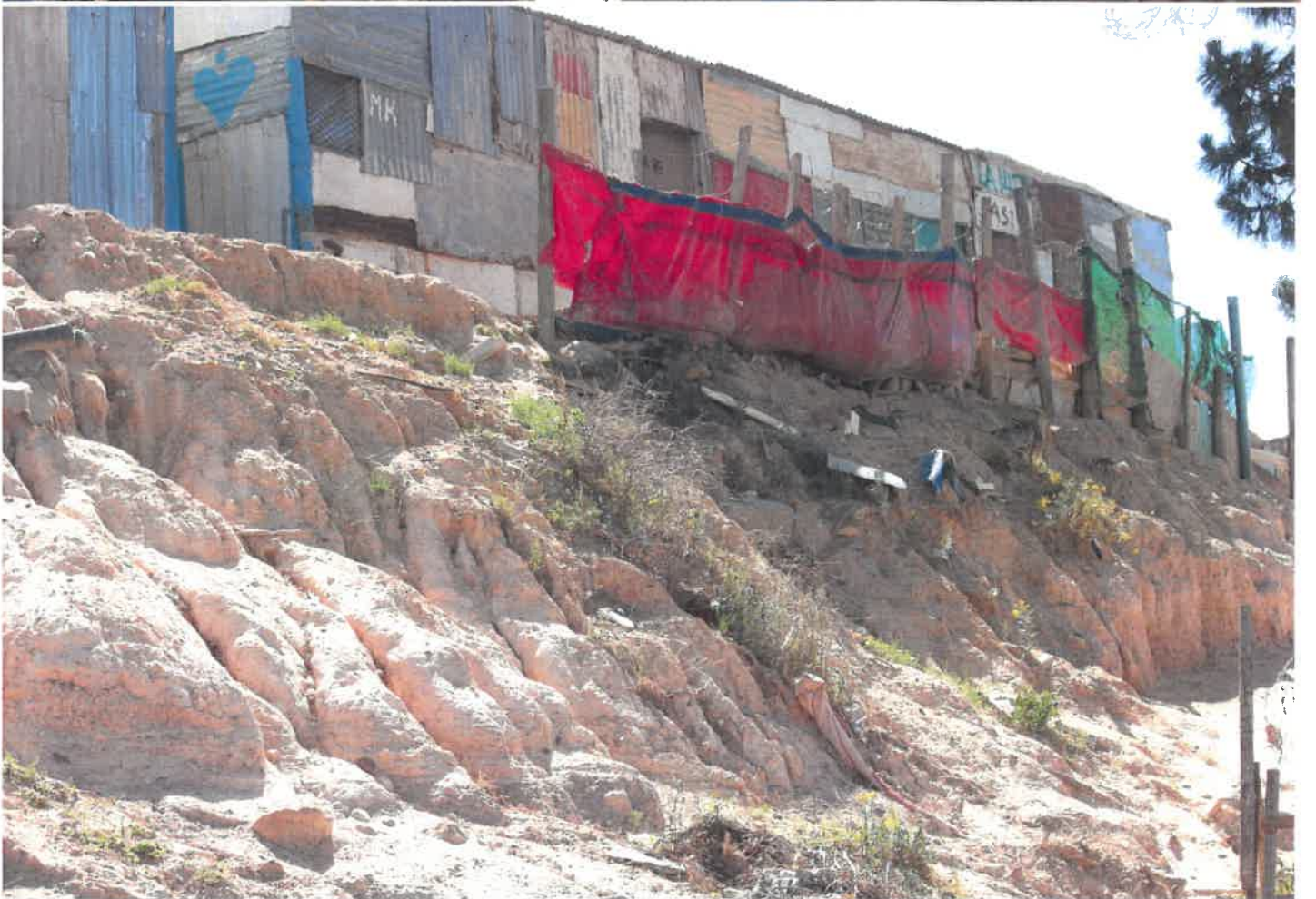
The dam site in Langrug
