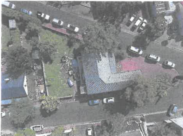
PHOTO 1: ERF 230, FRANSCHHOEK – AERIAL VIEW FROM ABOVE
