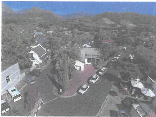
PHOTO 3: ERF 230, FRANSCHHOEK – ANGLED AERIAL VIEW FROM THE FRONT OF THE EXISTING BUILDING
