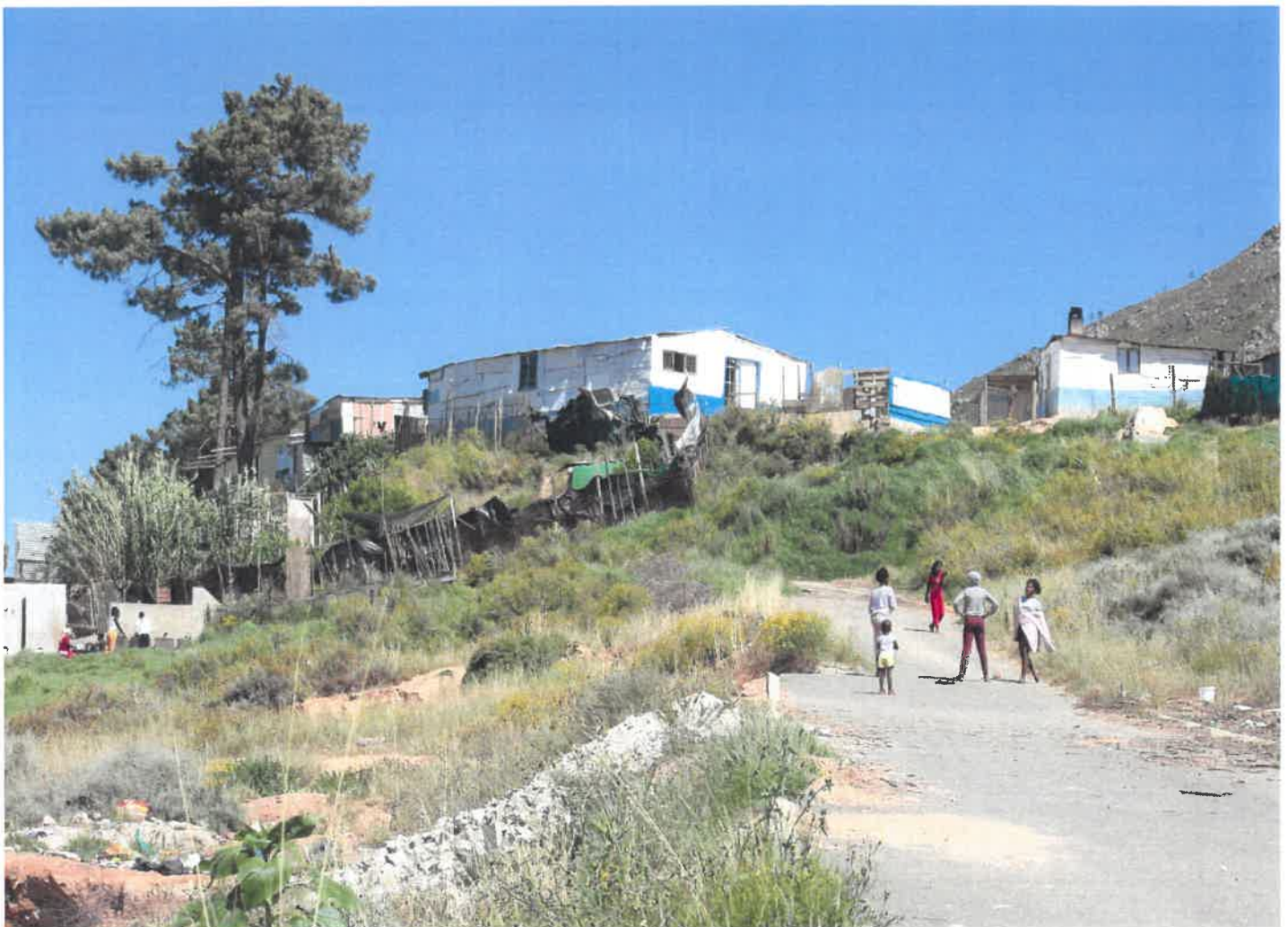
Structures on the dam-wall in Langrug
