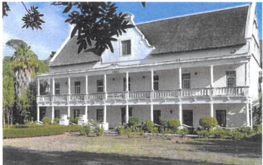
Fig 22 Existing Manor House
