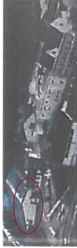
Figure 9: The Oude Molen site prior to the 1990 redevelopment (Architect & Builder March 1990), there is no visible plaster trademark embellishment on the Vinlab warehouse. A pergola and additional openings were subsequently added to the front facade.
