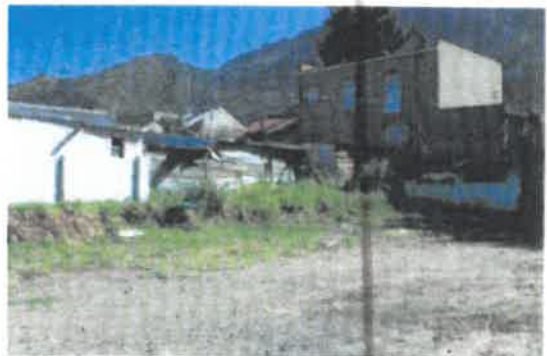
PHOTO 15: VIEW FROM ERF 2235 PARKING AREA TO ADJACENT ERVEN 2227 & 2228 (RESIDENTIAL)
