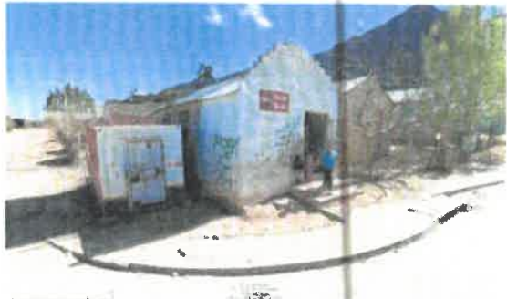
PHOTO 17: ERF 1993 (RESIDENTIAL & SHOP)
