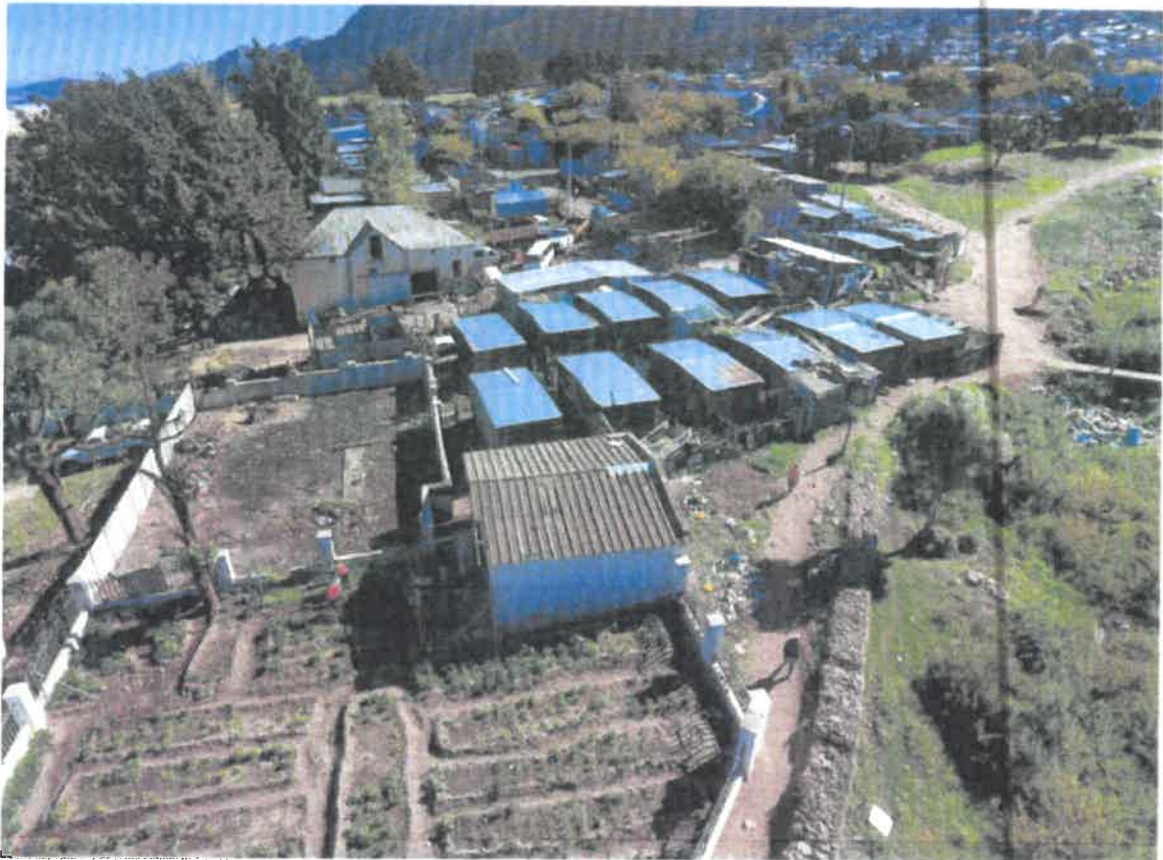
PHOTO 9: VIEW OF OTHER BUILDINGS FROM THE EAST
