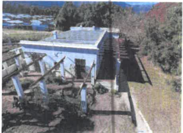
PHOTO 6: MAIN ACCESS TO EXISTING MAIN BUILDING
