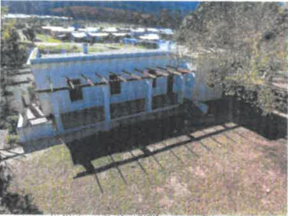
PHOTO 7: EXISTING MAIN BUILDING FROM THE SOUTH
