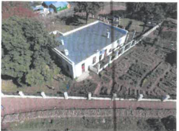
PHOTO 8: EXISTING MAIN BUILDING FROM THE EAST
