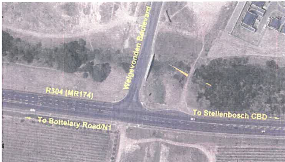
Photo 2 : Existing R304/Welgevonden Boulevard intersection lane layout
