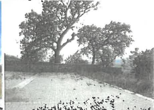
Internal road on Mentoer Estate to connect
