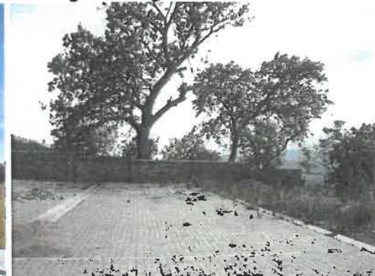
Internal road on Mentoor Estate to connect
