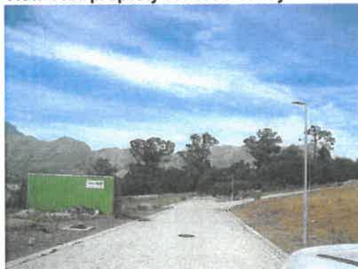
Existing access road to be extended
