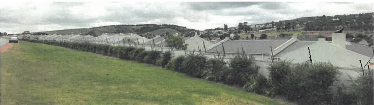
Photograph 6 Mount Simon housing development directly opposite the site, on the other side of the R304.
