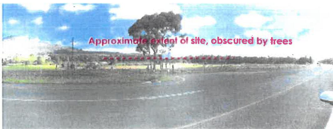
Photo Plate 6: View towards the proposed site of development, 1,8 kms east of the site. The existing trees in the mid ground of the photos will obscure the proposed Light Industrial Development
