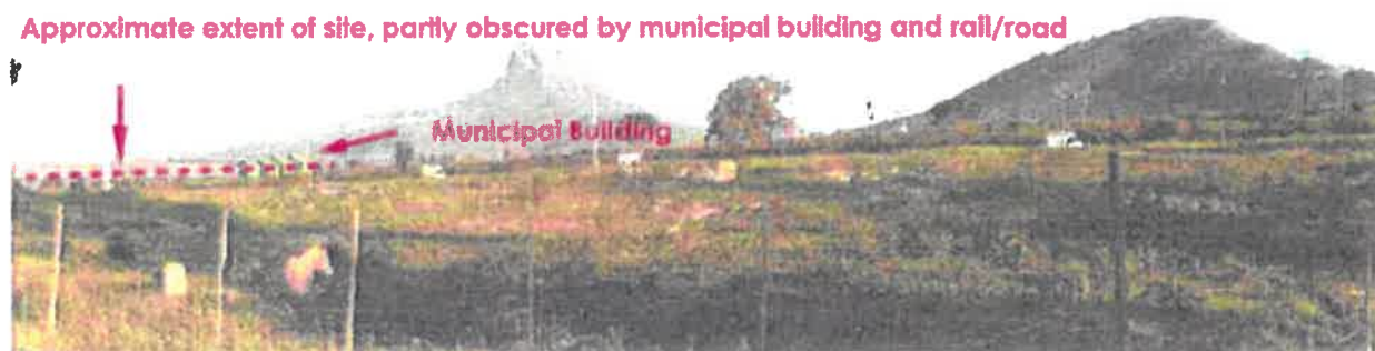
Photo Plate 9: Photograph taken from the N1 north west of the site. Proposed site and buildings will be behind the green municipal building
