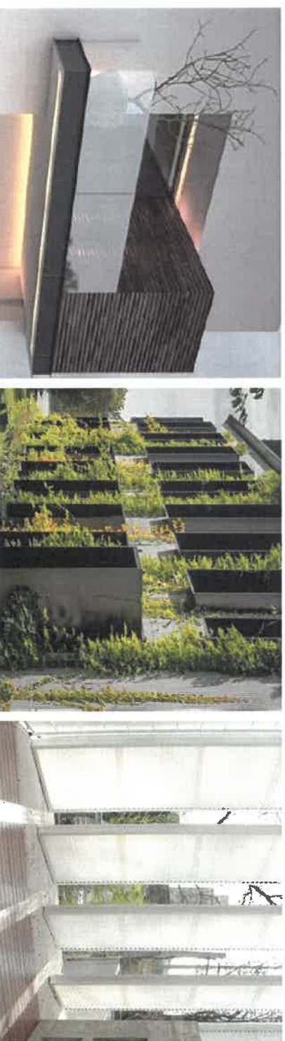
Figures 112- 118: Image showing facade shading through planting and louvers, deep recesses, colonnades, balconies, eaves and overhangs
