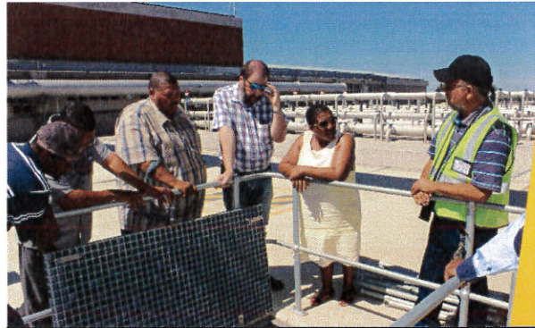
MPAC/Oversight visit Devon Valley WWTW R400 million project
