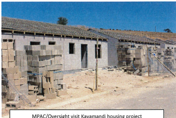
MPAC/Oversight visit Kayamandi housing project
