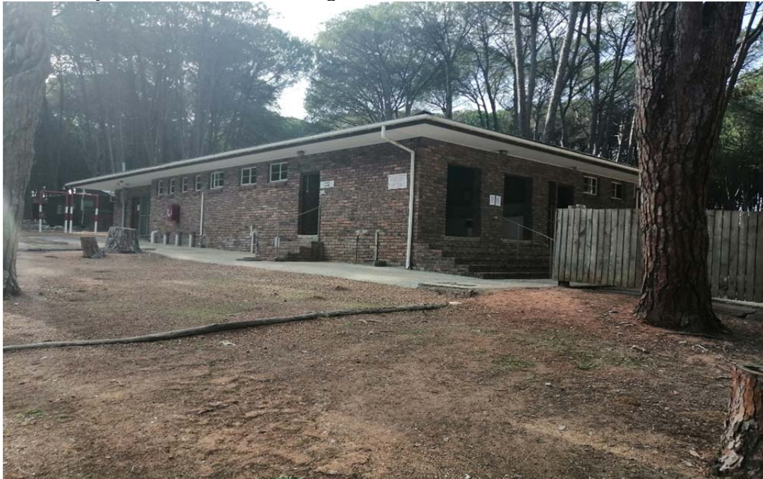
Fig 19: Main ablution facilities
