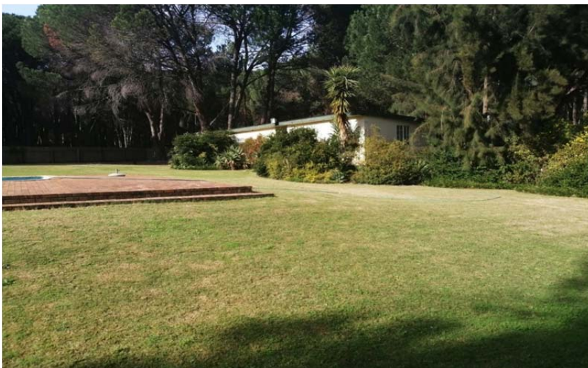
Fig 18: Swimming pool and ablution facilities
