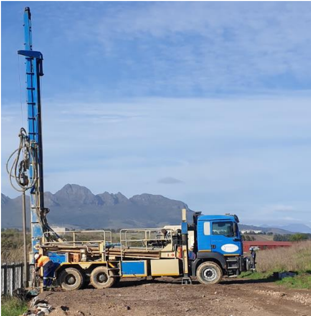
Photo: Drilling of well on-site
