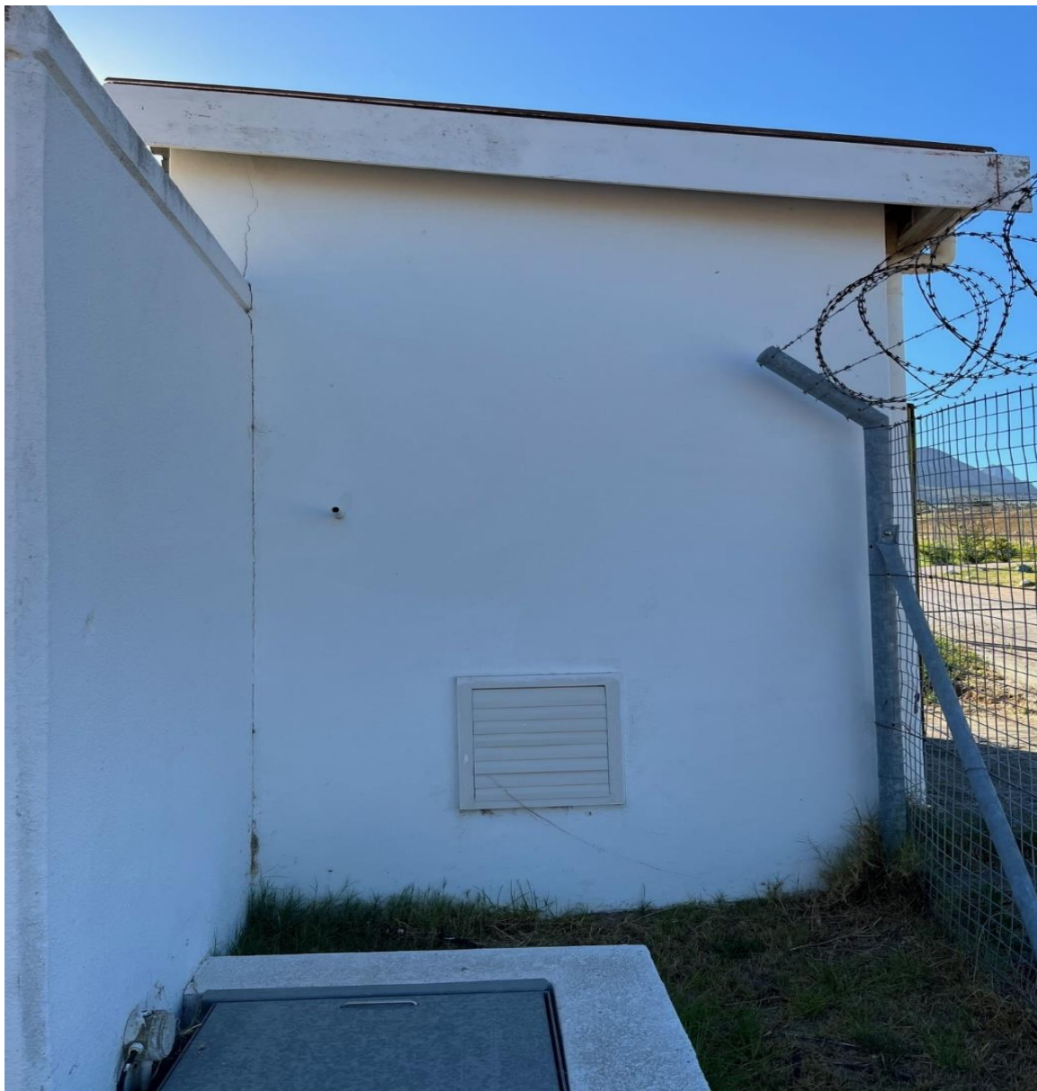
Figure 4: Outer wall of extractor showing louvres.
