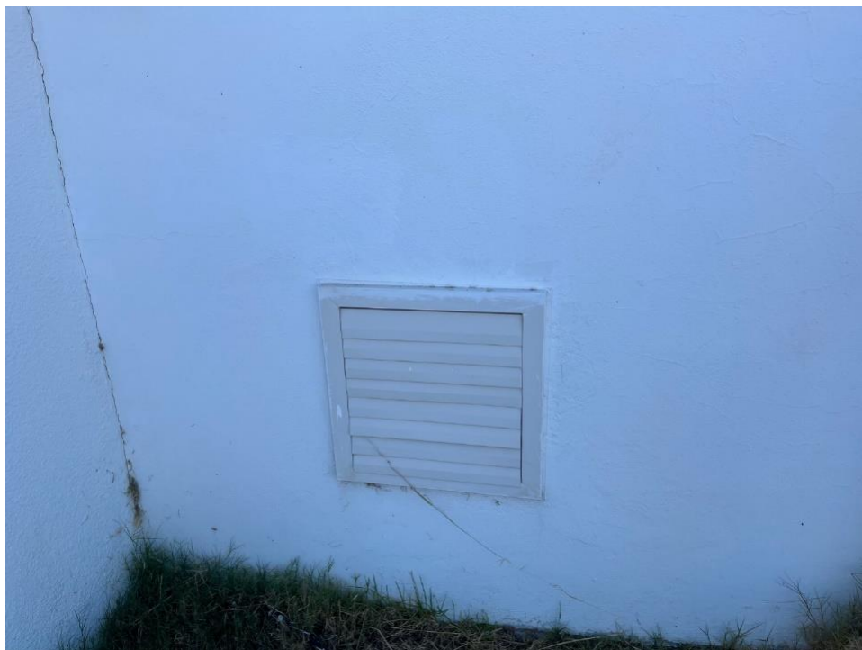
Figure 2: Extractor Fan Outer Louvres
