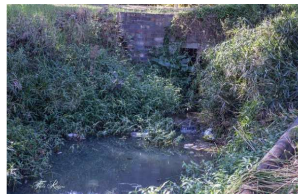
Figure 9: Water quality and habitat diversity in the Plankenbrug River have been reduced by stormwater and wastewater discharges from Kayamandi and Stellenbosch. This river has been identified as a high risk area for human health
