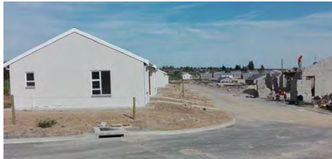
Figure 51 Construction in process
