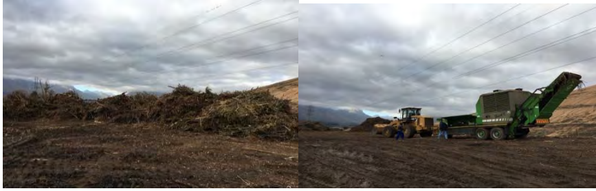
Figure 18 Shredded greens & Shark shredder used on site
