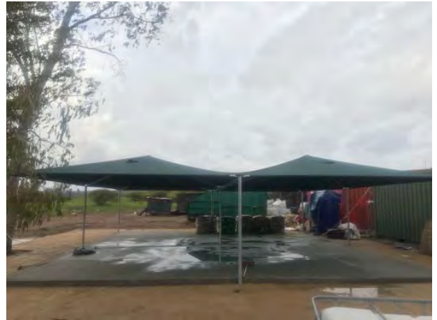
Figure 25 Preparation work for second slab
