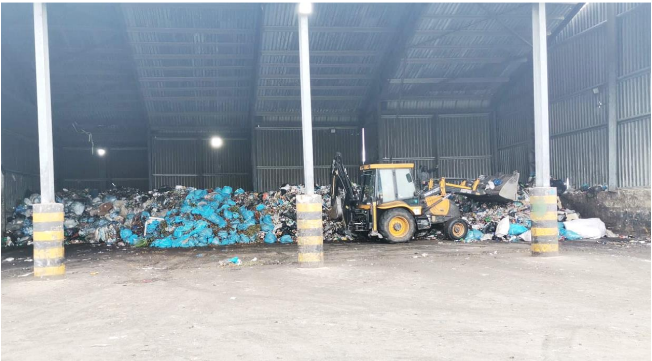
Photo: Klapmuts Transfer Station
