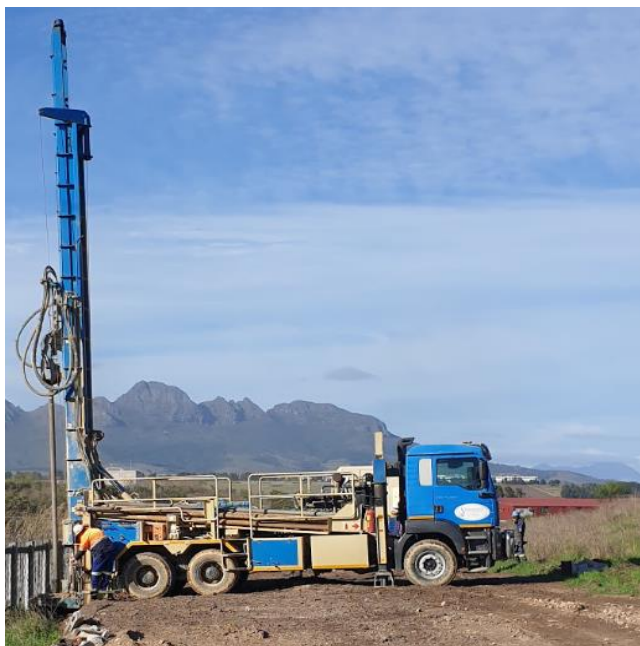
Photo: Drilling of well on-site
