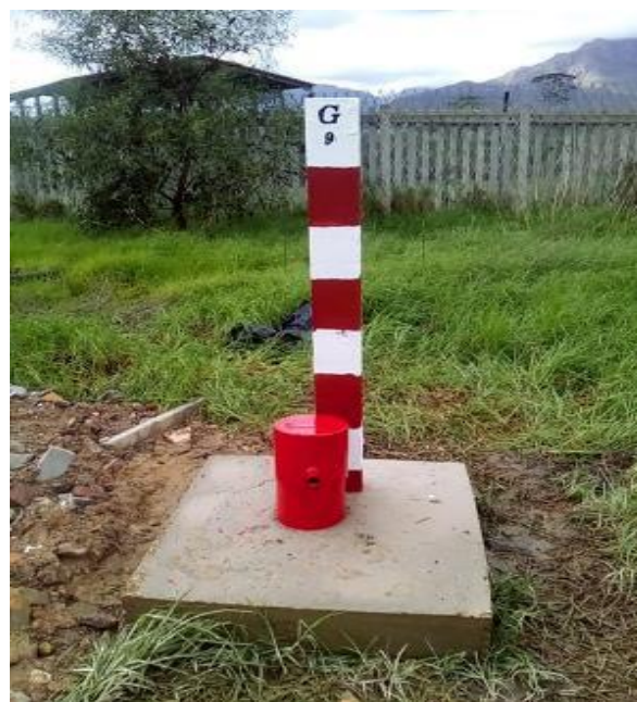
Photo: One of the installed gas monitoring wells
