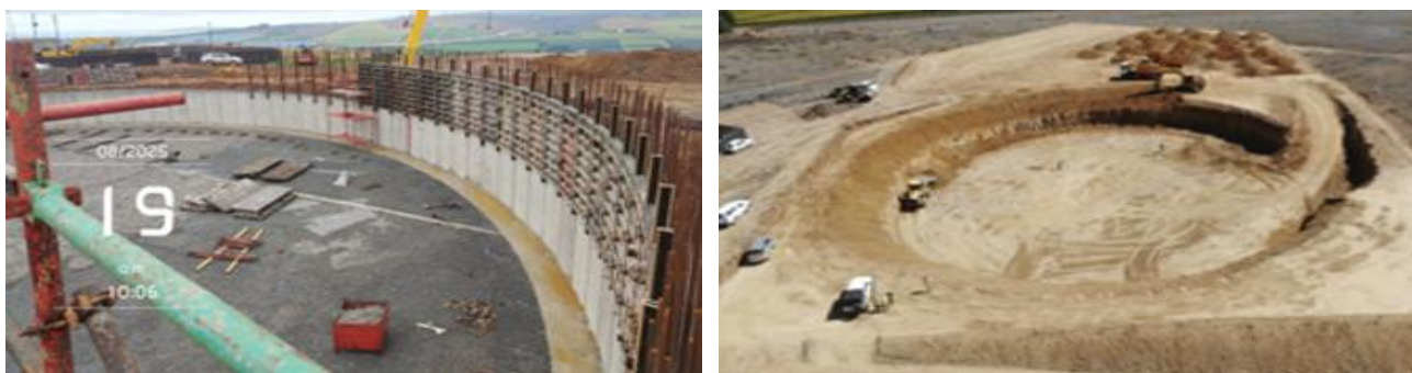
Image 20: Construction progress of the Stellenbosch 10ml Reservoir, Bulk Water Supply, and Associated Works
