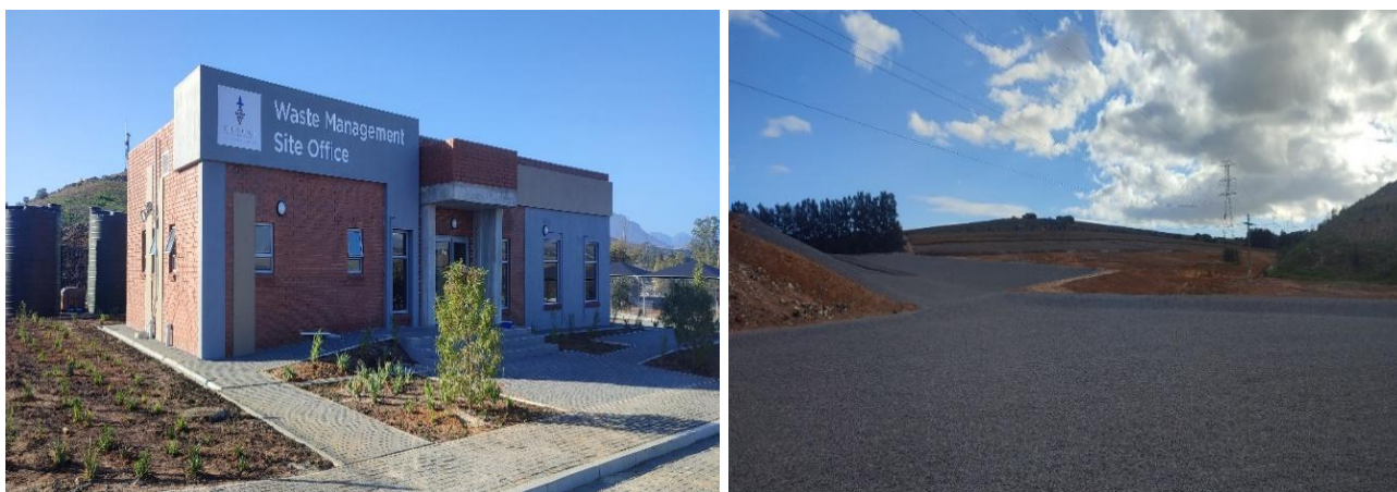
Image 21: Stellenbosch Landfill - Construction of New Assets
