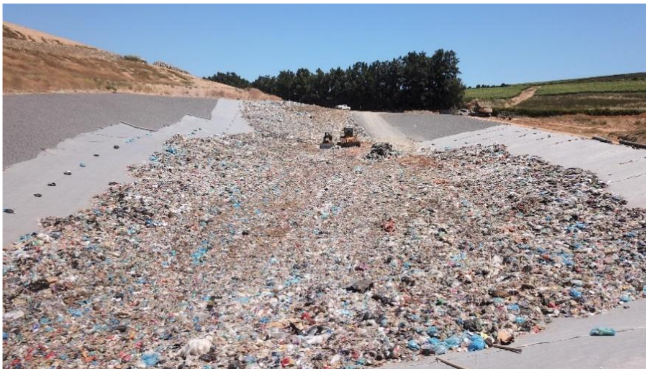
Image 5: Cell 4A at the landfill site
