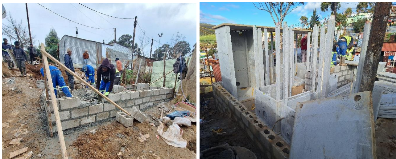
Image 7: Construction of ablution facilities in Enkanini, Kayamandi
