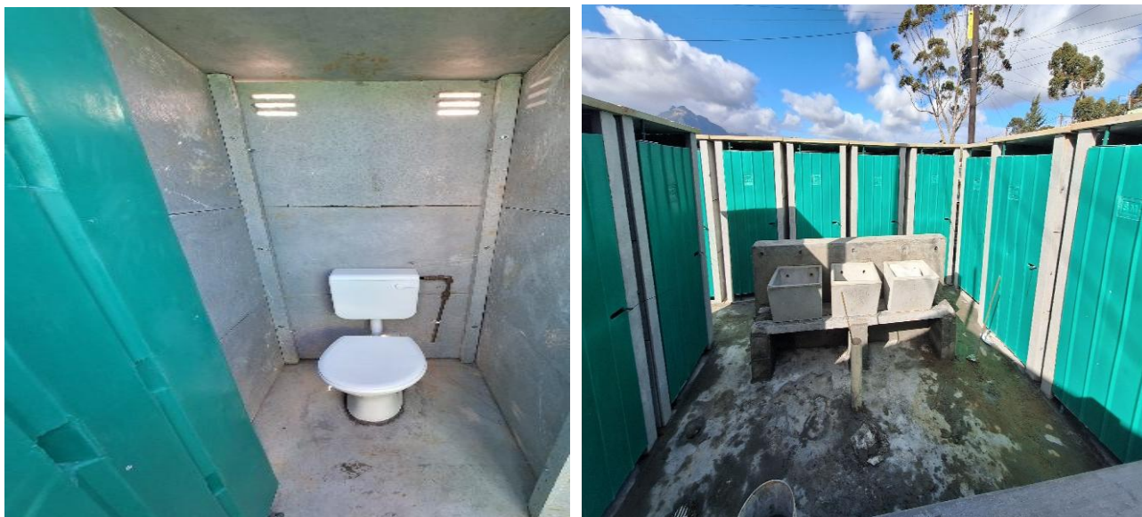
Image 8: Completion of ablution facilities
