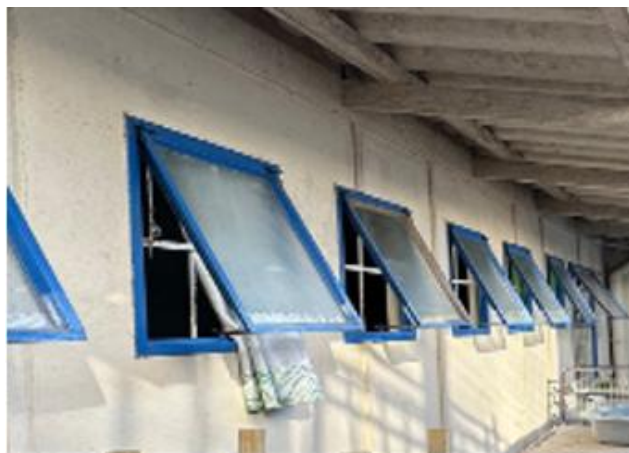
Image 16: Upgrading of Municipal ECD Facilities
