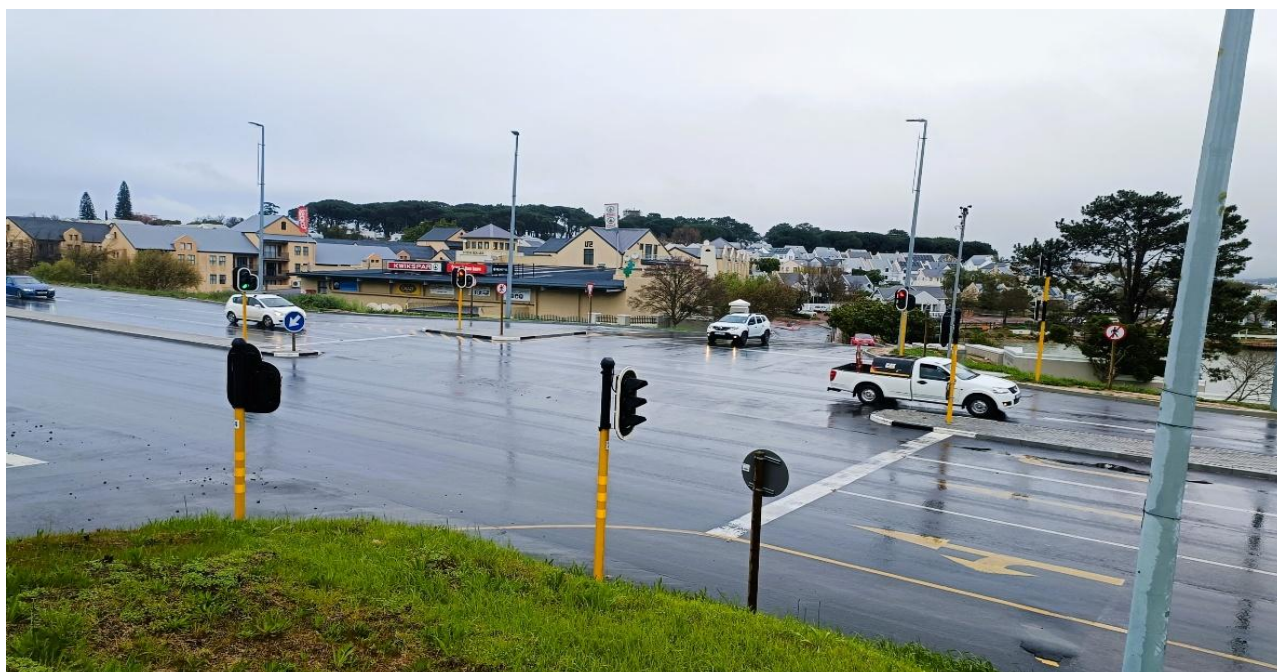
Image 26: Upgrading of R44 / Hendrickse Street (Cloetesville)
