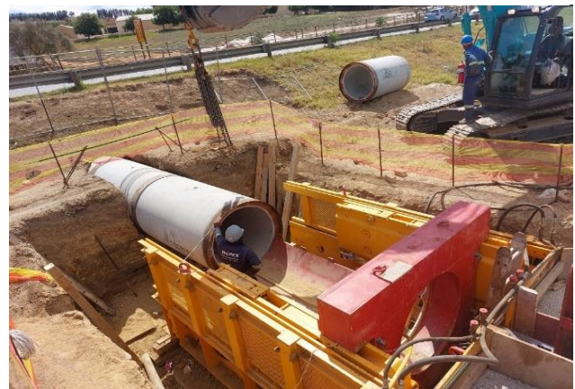
Figure 47: Outfall Sewer upgrade (Newinbosch)
