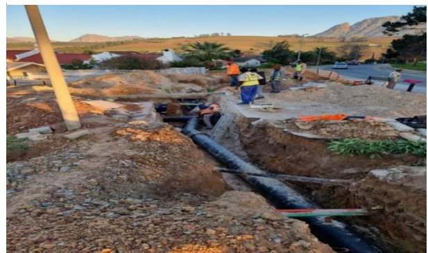
Figure 43: Vlottenburg New Outfall Sewer (Longlands)
