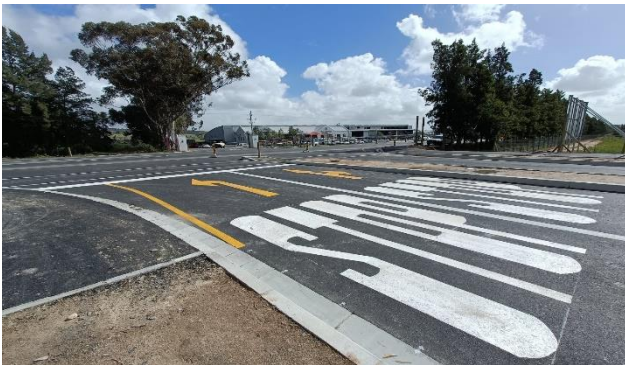
Figure 42: Klapmuts Road intersection Upgrade
