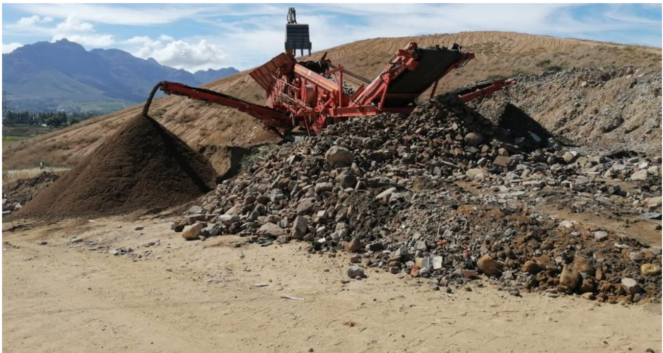
Figure 16: Crushing of builders rubble done on site
