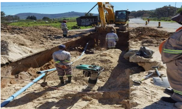
Figure 44: Cloetesville Bulk water upgrade (Voliere)
