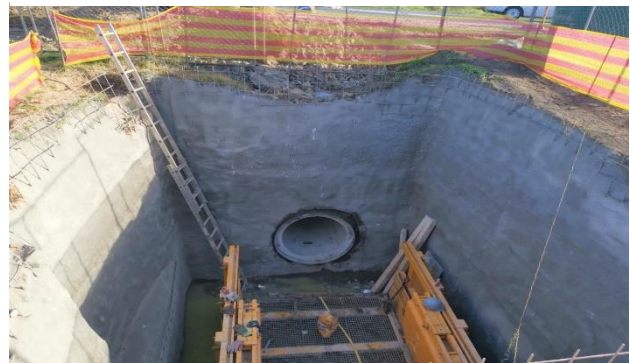
Figure 41: Sewer Crossing Bottelary Road (Devonbosch)
