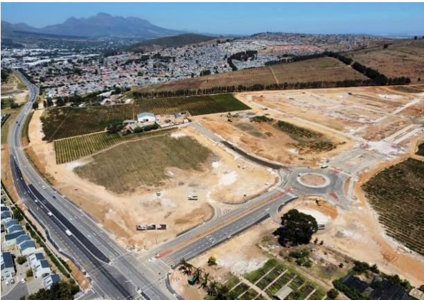
Figure 46: R304 intersection upgrade (Newinbosch)
