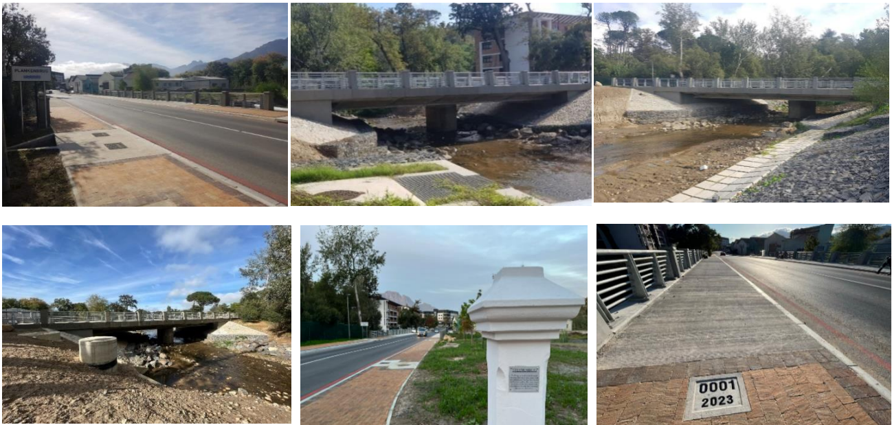
Figure 32: New Bridge constructed
