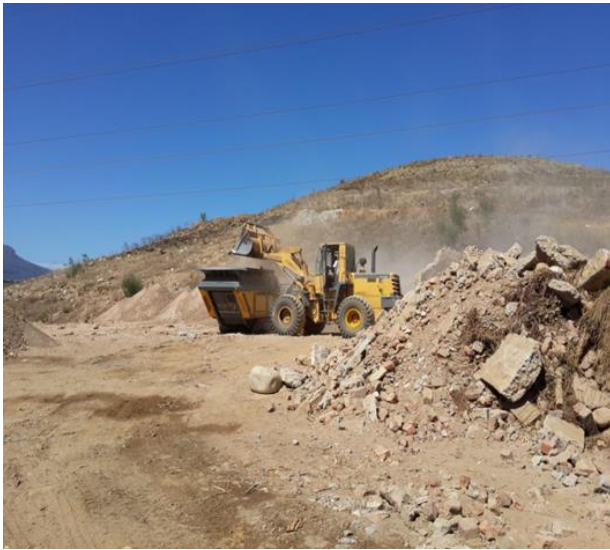
Stellenbosch Landfill rubble crushing and landfill side slope rehabilitation
