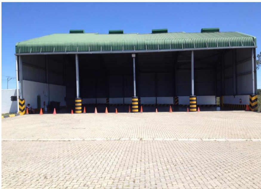
Klapmuts Transfer Station waste reception apron
