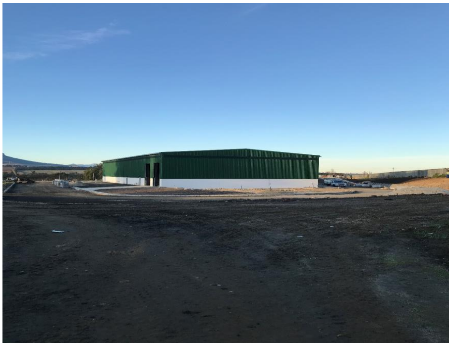
New MRF building under construction
