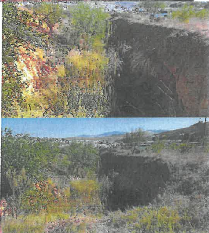
Right and bottom photo showing scale of "detention pond", approximately 3m deep, 5m wide and 30 m long.
