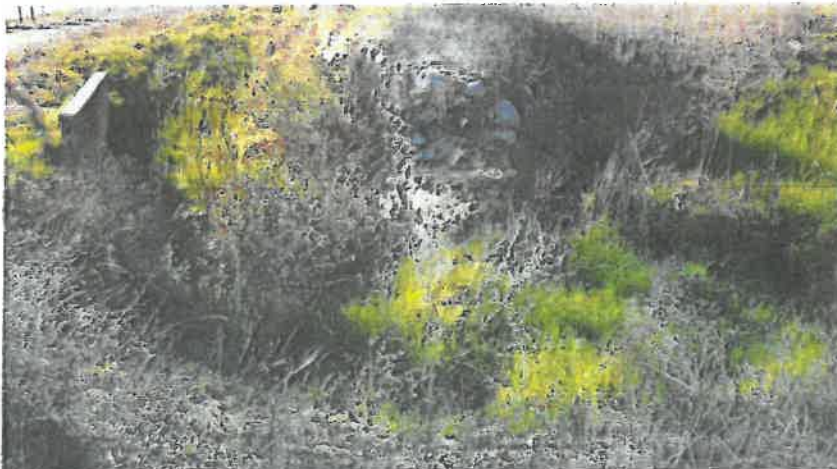
Drainage structure measuring some 8 x 8 m and a depth of 4m with a water current deflector wall. This large structure also serves as a detention pond before the water dissipates into the wetland area.
