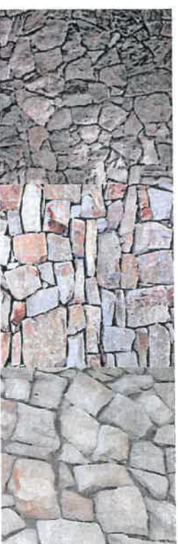
figure 6: Allowed stone cladding construction
